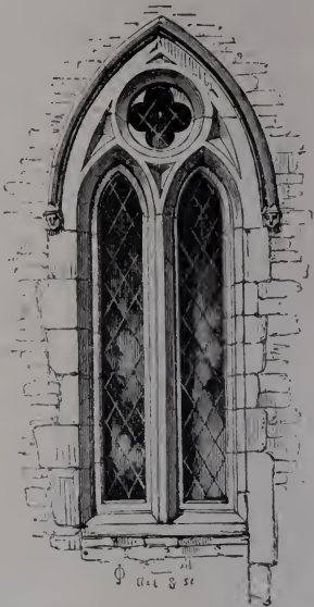
91. Charlton-on-Otmoor, Oxon., c. 1240. Shewing a window of two lights with a quatrefoil in the head of plate-tracery, and a dripstone terminated by the characteristic ornament called a mask or a buckle.
