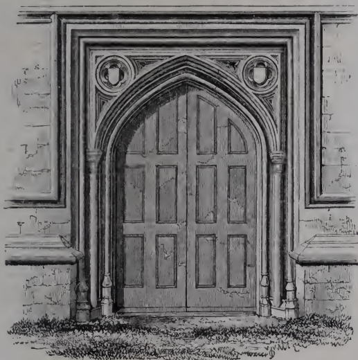
151. Fotheringhay, Northamptonshire, A.D. 1440.
