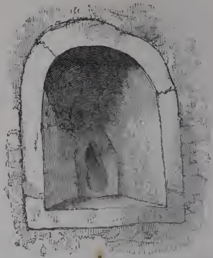
10. Window, Caversfield, Buckinghamshire, With small opening and very wide splay.
