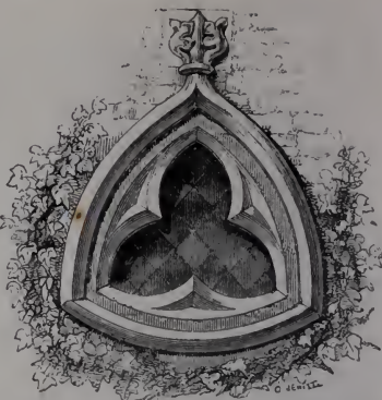
126. Cranford St. Andrew, Northants., c. 1320. Clear-story Window of the form called a spherical triangle.
