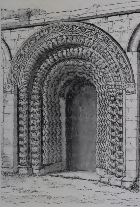
32. West Doorway, Ifley Church, Oxfordshire, c. 1160.
