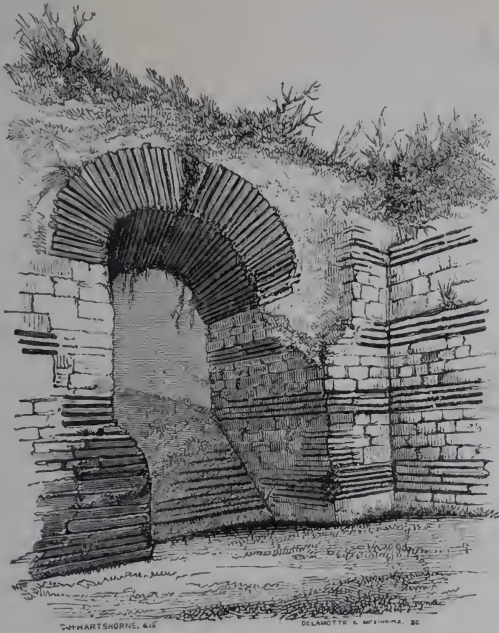
1. Porchester Castle, Hampshire. Roman Masonry and Arch formed of Roman bricks or tiles.
