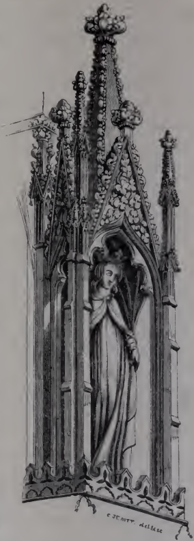
136. Open Niche, with Canopy and Pinnacles, and Figure of Queen Eleanor, from her Monumental Cross at Northampton, A.D. 1294.
