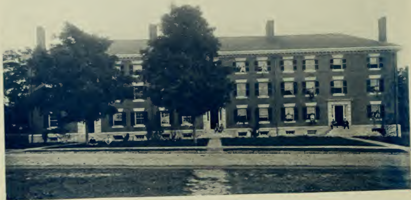
BANCROFT COTTAGE, PHILLIPS ACADEMY.
