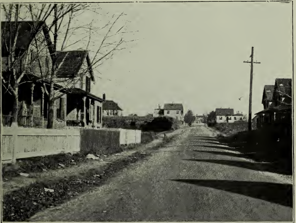
CLARENDON AVENUE.—After Construction.
