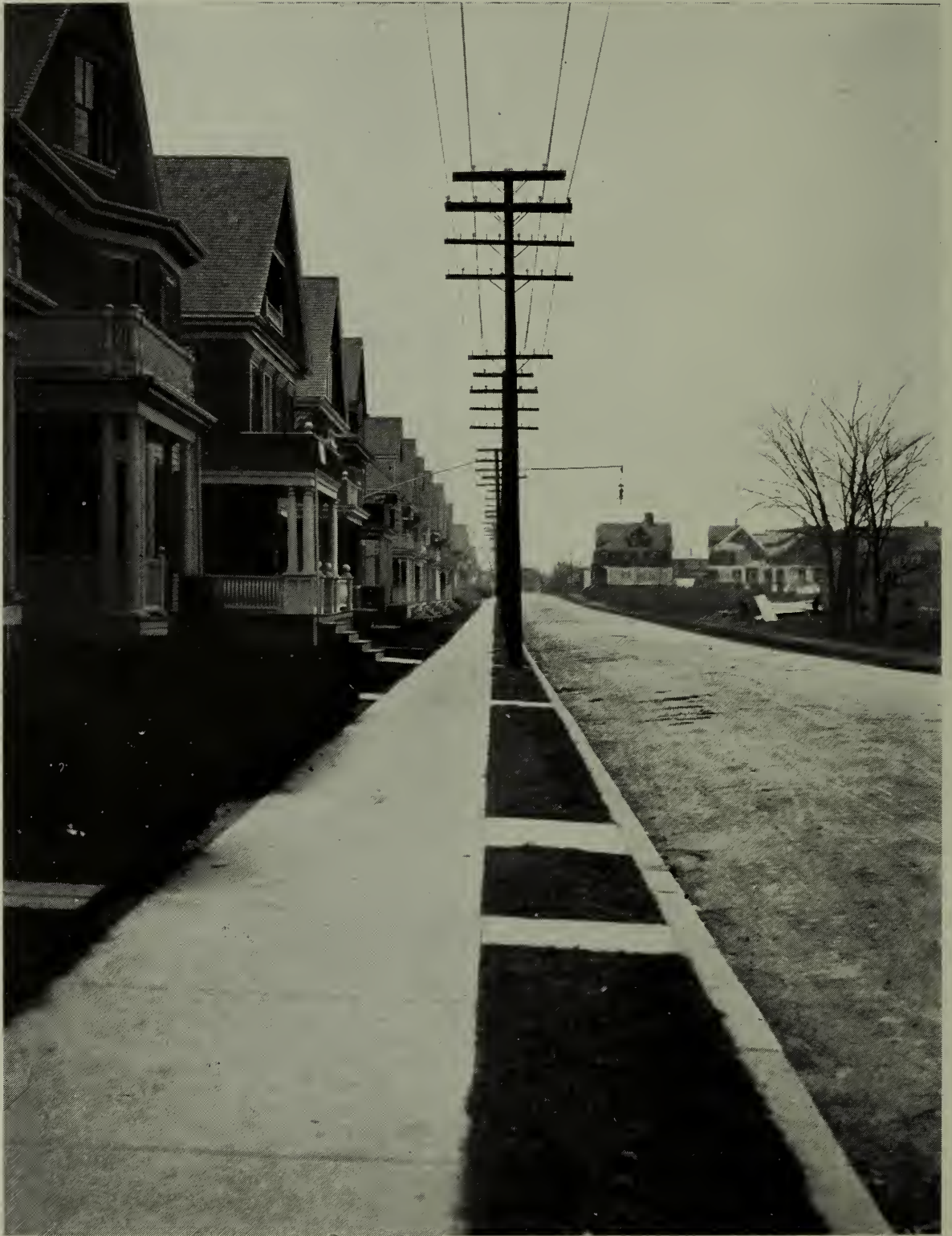
WILLOW AVENUE. Granolithic Laid by Highways Department.
