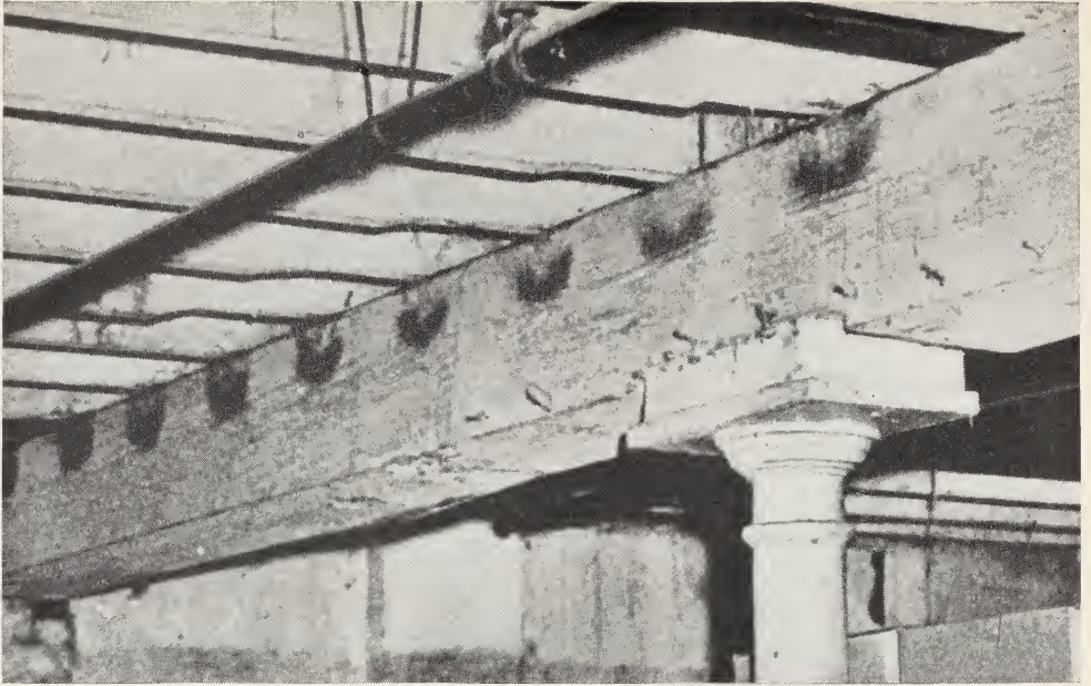
Fig. 5.—Smears made by rats traveling along a supporting floor beam. The rats must crawl along the side of the beam under each joist, and thus leave the U-shaped markings. Courtesy of U. S. Public Health Service.
