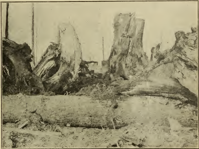
FIG. 8.—The result of a battery shot upon the stumps shown in figure 7.
