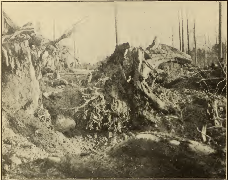
FIG. 9.—Two stumps, similar to the ones shown in figure 7, that were shot by the fuse method. The stump upon the left was not thrown out, as the charge under the right-hand stump exploded first, destroying the effect of the charge under the stump upon the left.
