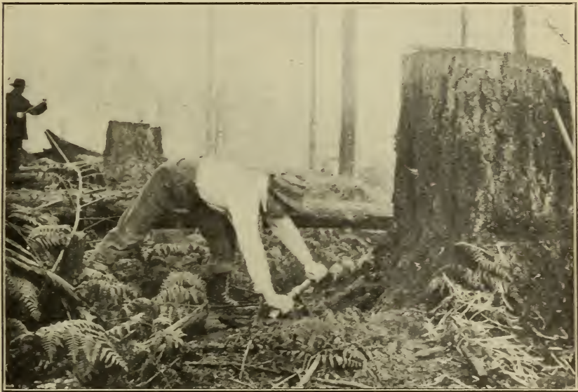
FIG. 6.—Finishing the boring of holes under a stump for blasting.
