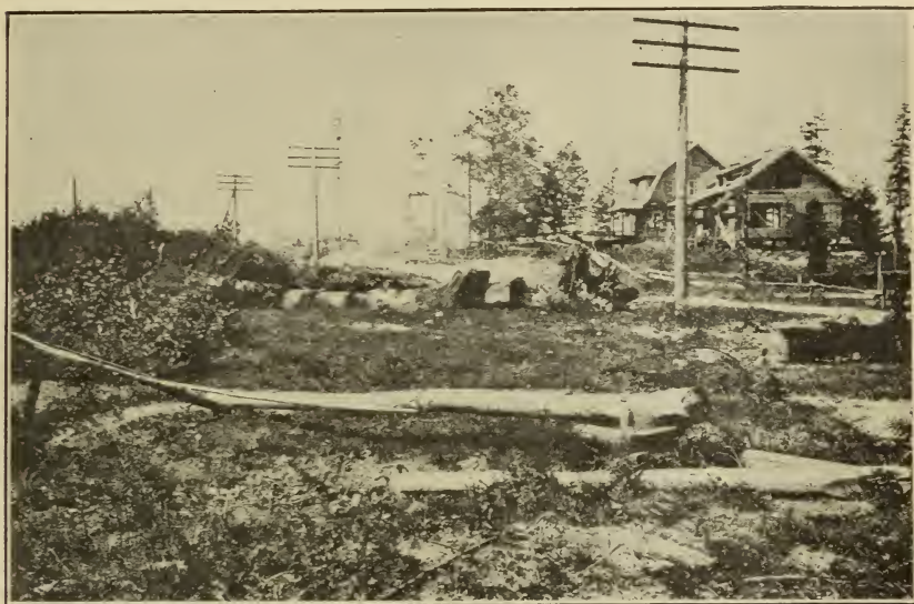
FIG. 10.—The simplest form of a stump puller. This pulls the stump to the side. It is operated by one man and a horse.
