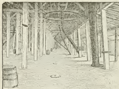
Fig. 512. View of the interior of a large terminal elevator, showing the spouts leading from the scale hoppers on the floor above to the bins below.
