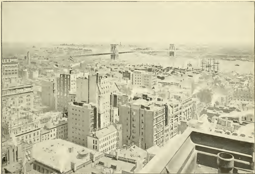
VIEW LOOKING NORTHEAST FROM ROOF OF OFFICE BUILDING, 66 BROADWAY.
