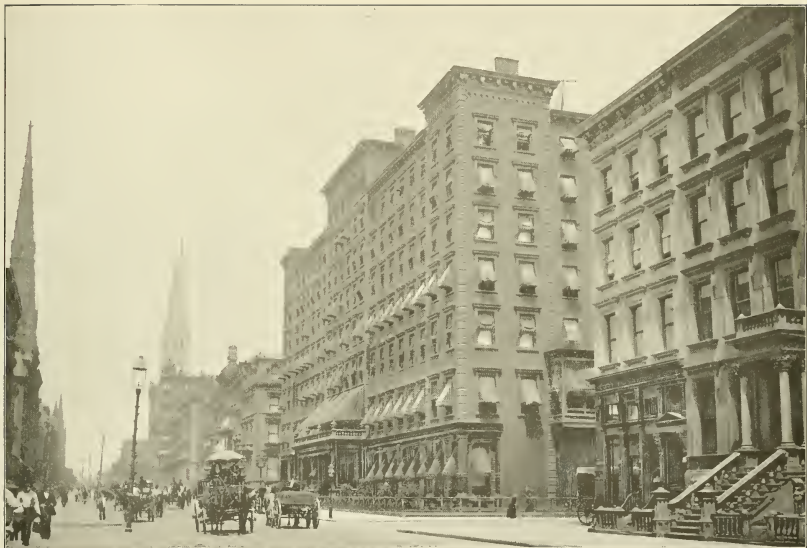
WINDSOR HOTEL AND FIFTH AVENUE — Looking North from Forty-sixth Street.
