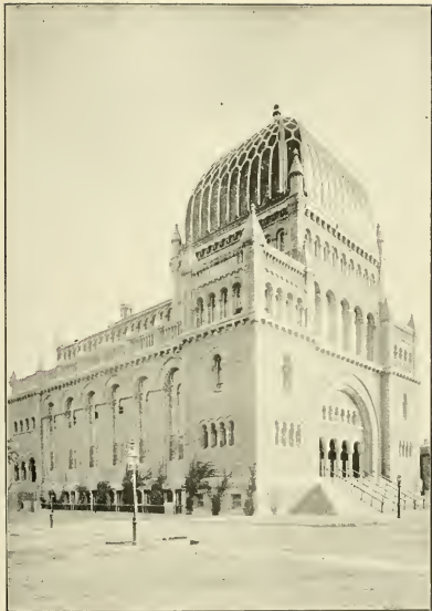
TEMPLE BETH-EL, HEBREW — Southeast Corner Fifth Avenue and Seventy-sixth Street.
