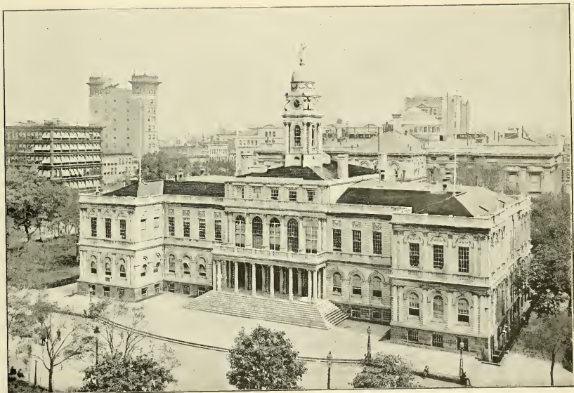
THE CITY HALL, NEW YORK—In City Hall Park, between Broadway and Park Row, opposite Murray Street.
