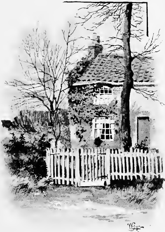
OLD COTTAGE IN WILLESDEN LANE
