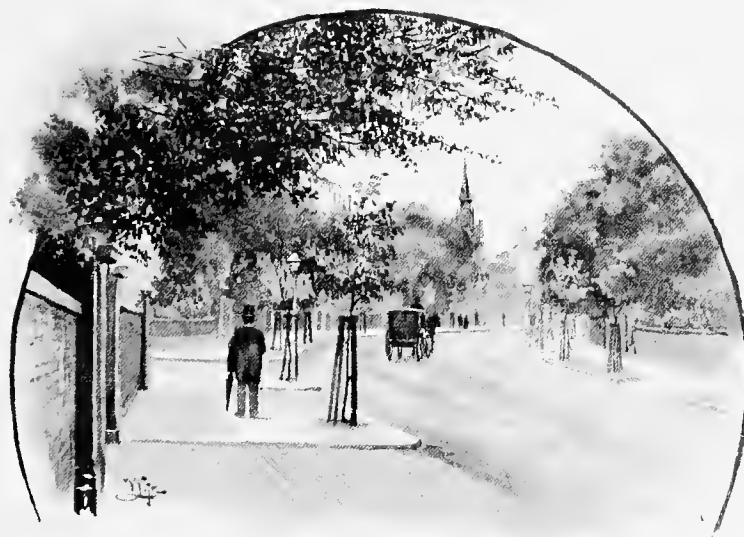
AVENUE ROAD, ST. JOHN'S WOOD
