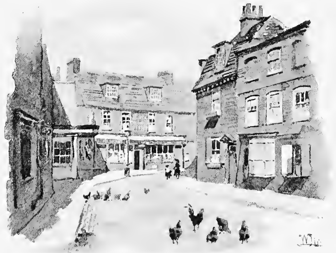
CHURCH STREET, CHISWICK
