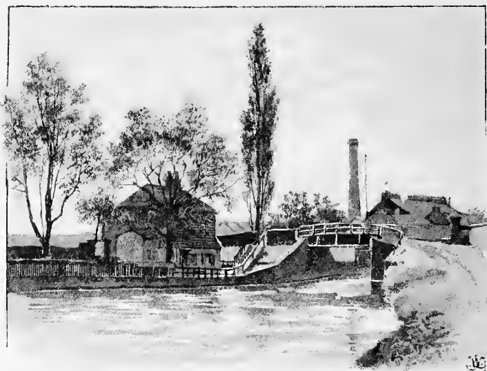
NEAR LEA BRIDGE
