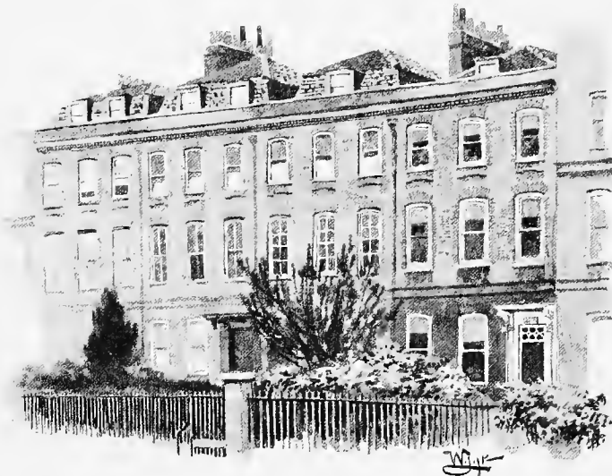
OLD HOUSES AT CLAPHAM COMMON, NORTH SIDE
