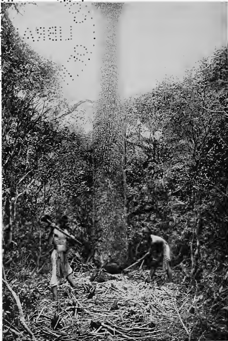
TIMBER FELLING IN THE CHACO.
