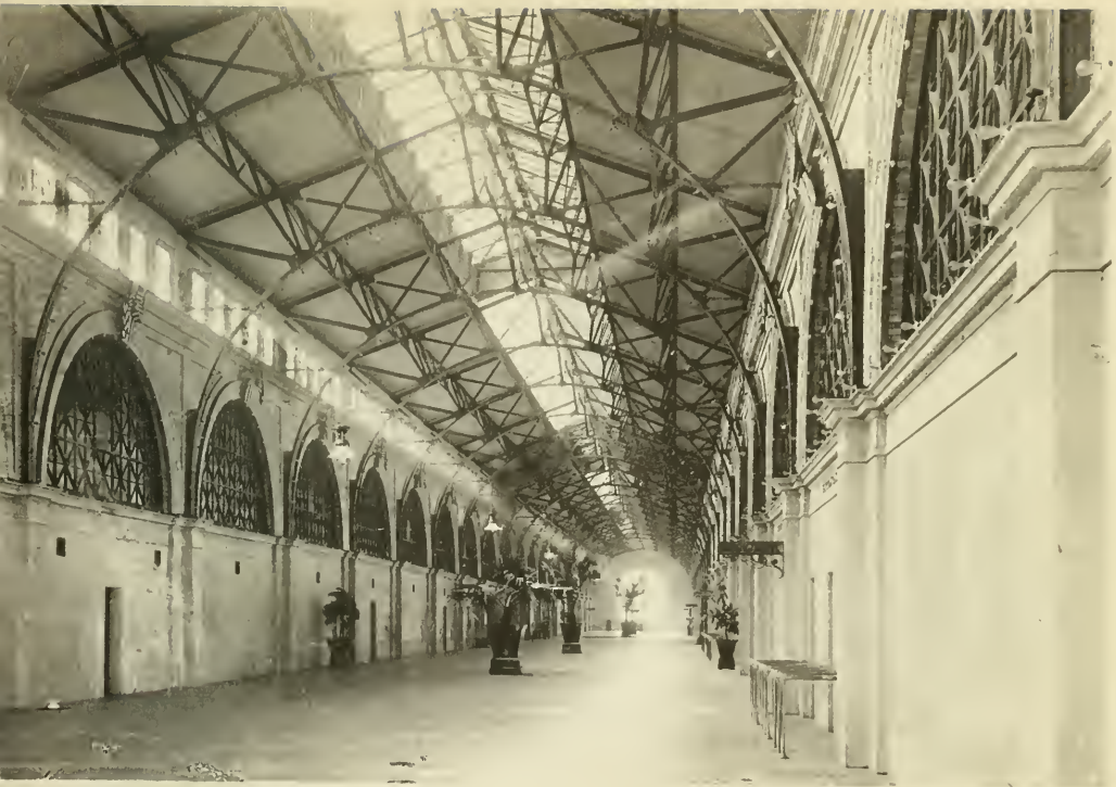
UPPER CORRIDOR—FERRY BUILDING.
