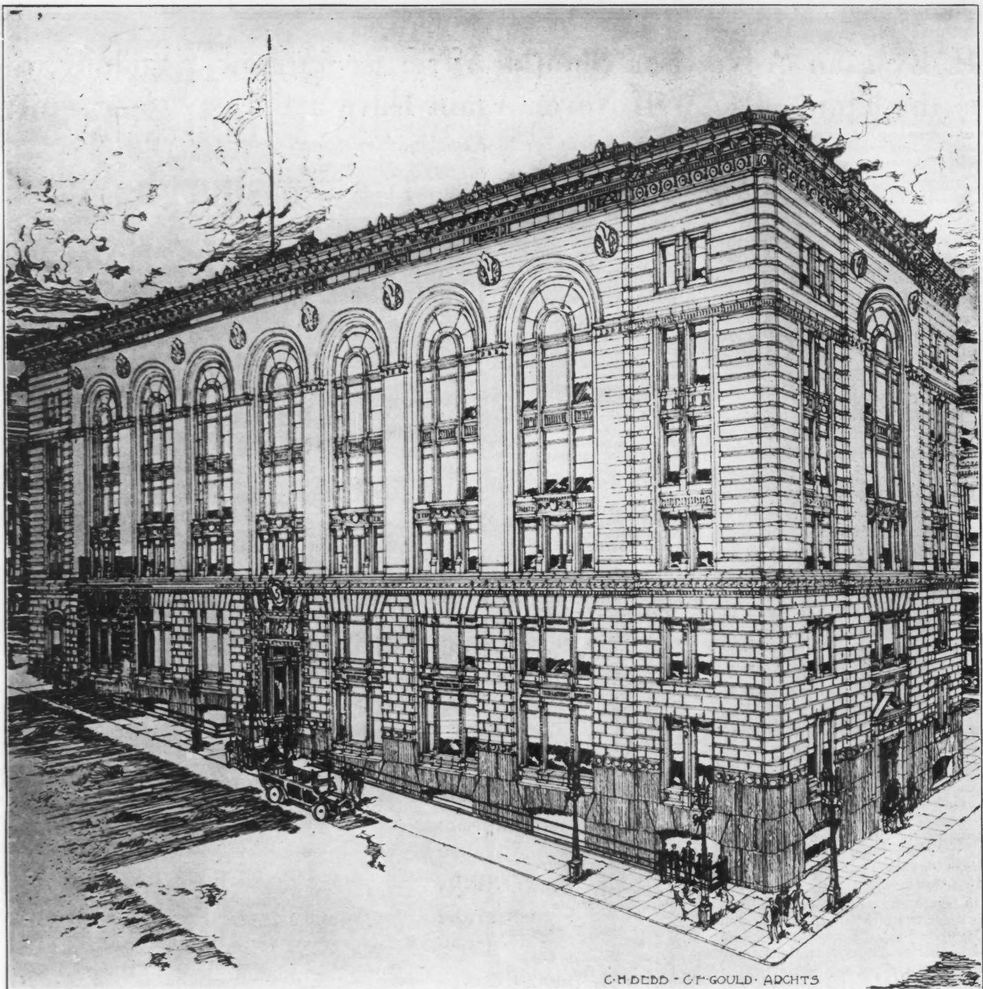
NEW HOME OF THE SEATTLE TIMES, NOW UNDER CONSTRUCTION
