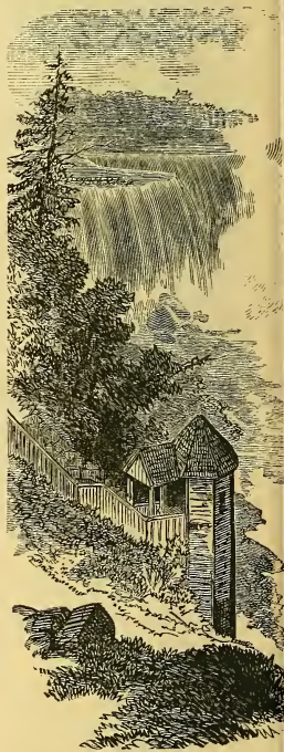
Biddle Stairs from above.
