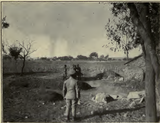
TSINGTAU ON THE MORNING OF OCTOBER 31
