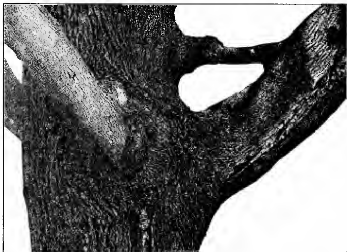
FIG. 104—LIVING WOOD BRACE BETWEEN TRUNK AND LIMB OF NORWAY MAPLE. SHOULD HAVE BEEN MADE HIGHER UP TO BE STRONGER
