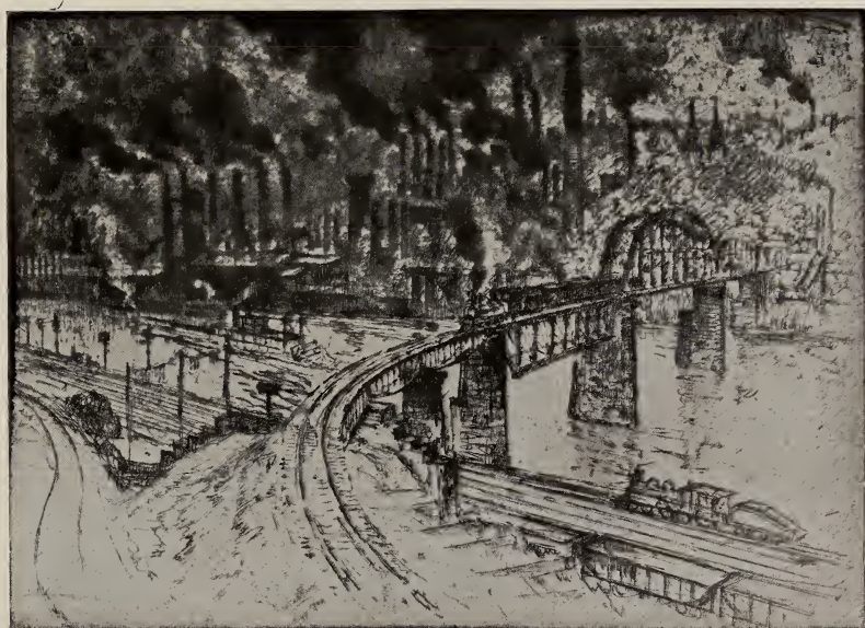
THE CURVING BRIDGE, PITTSBURGH
