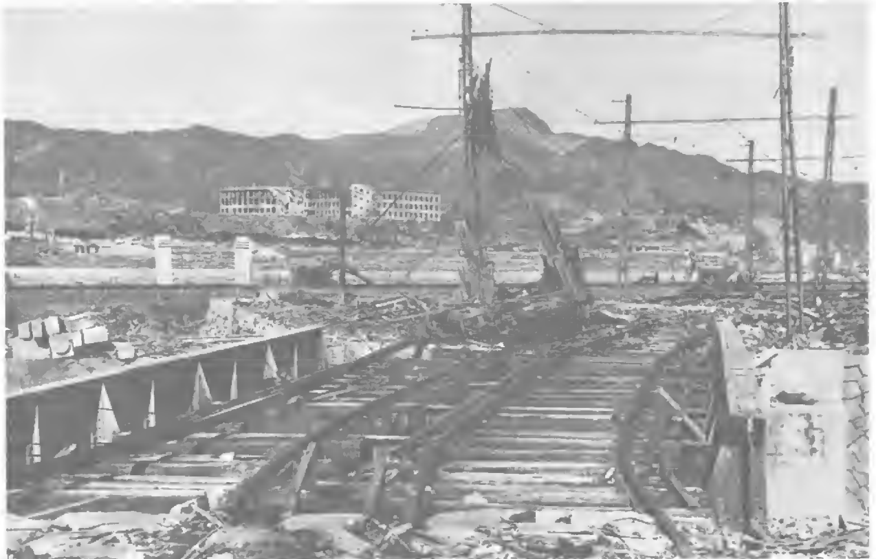
Figure 3-4. Structural Damage from a Nominal Airburst to a Steel Plate Girder Railway Bridge Located about 280 Yards from Ground Zero
