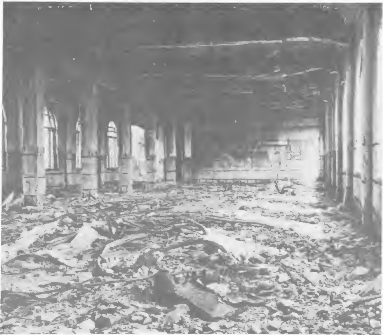
Figure 3-2. Interior of a Reinforced Concrete Building after a Nuclear Airburst
