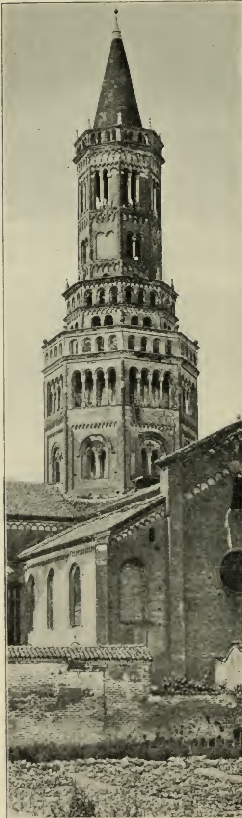
Fig. 88. Chiaravalle. Central Tower.
