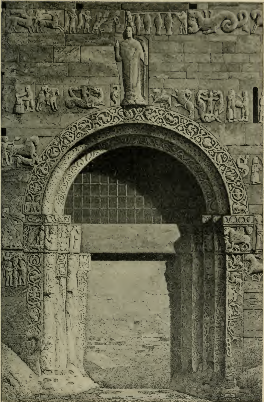
Fig. 127. S. Michele, Pavia. Right-hand Doorway of Façade.
