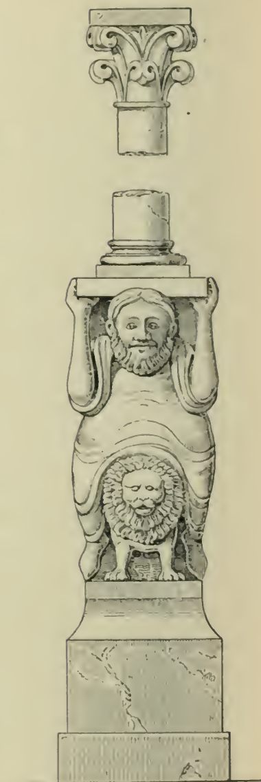
Fig. 135. Piacenza. From the Façade of Cathedral.
