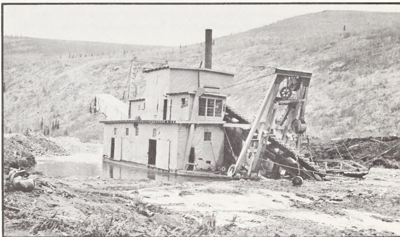
Typical placer mining dredge, located on Jack Wade Creek, circa 1920's. Photo courtesy of the Anchorage Museum of History and Art.
