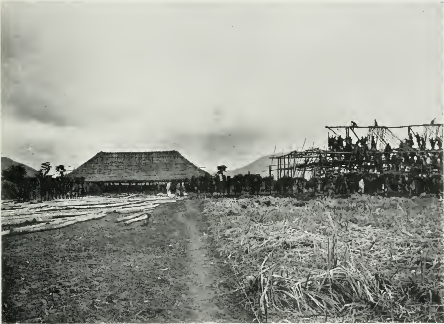
192. "GOVERNMENT HOUSE" AT HOIMA, UNYORO, IN PROCESS OF BUILDING
