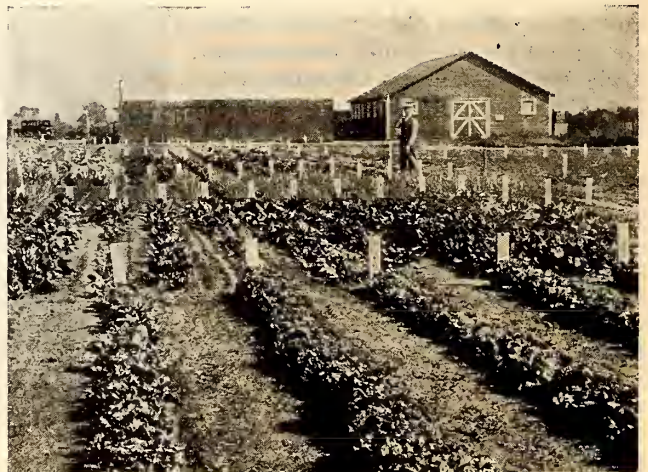
TESTING PLANTS AT ONE OF GERMAIN'S TRIAL GROUNDS
