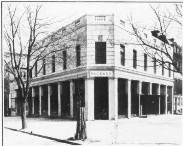
Packard salesroom, Washington, D. C. A good example of the use of Indiana limestone for small modern commercial buildings
