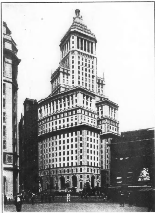
Standard Oil Co. Building, New York City, showing the use of Indiana limestone facing in large modern office building
