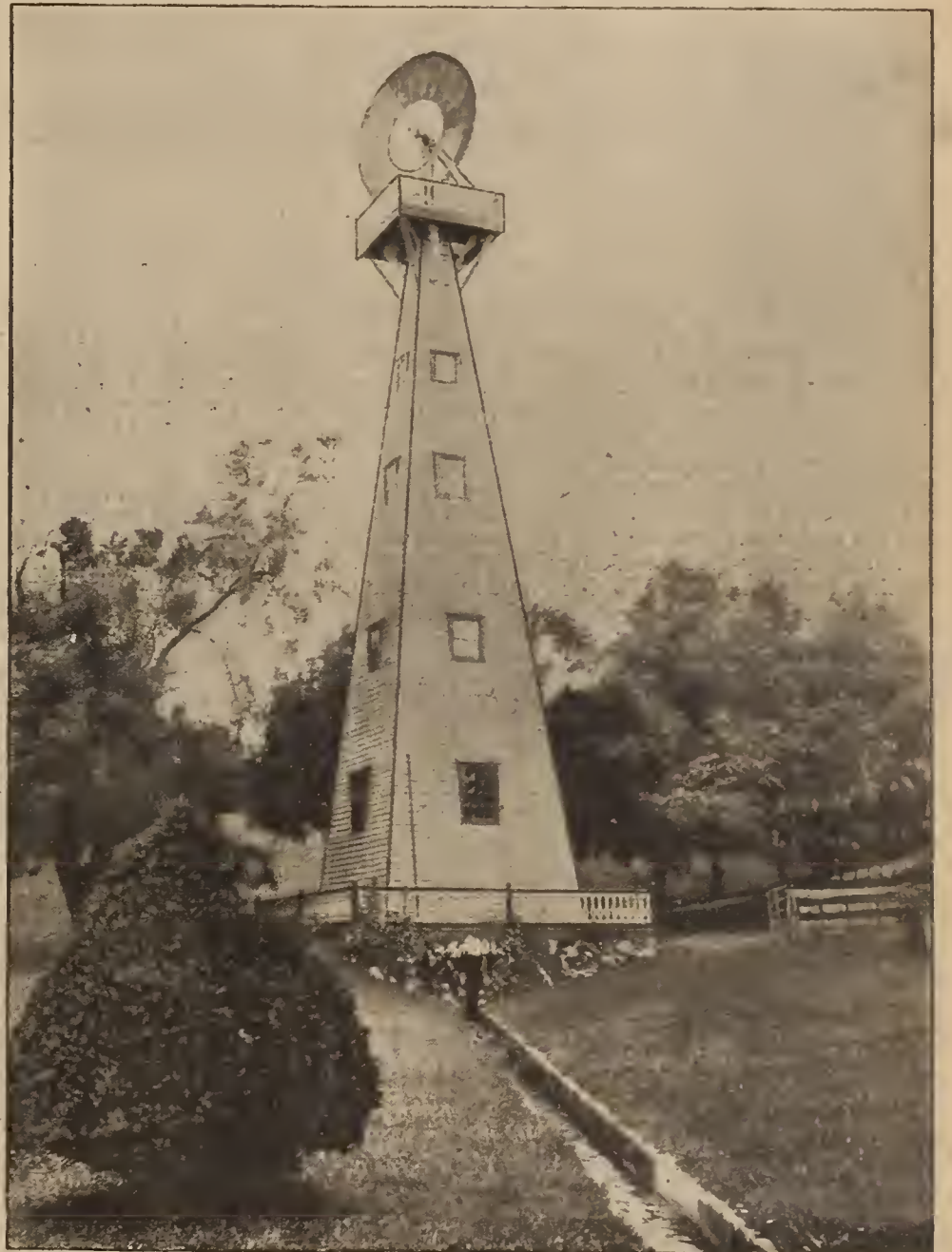
A CHARACTERISTIC TYPE OF THE INCLOSED WINDMILL HAS THE ENTIRE STRUCTURE BOARDED UP ON THE FOUR SIDES
