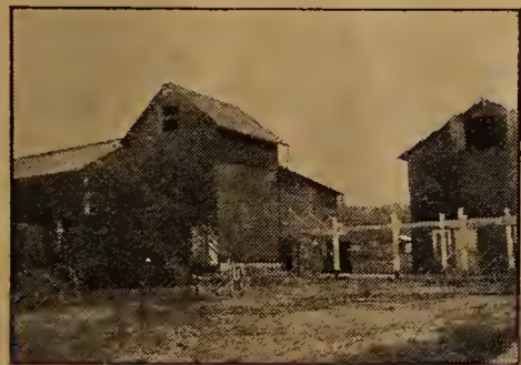
The first silo
