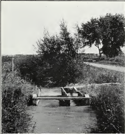
FIG. 2.—DIVISION BOX ON THE ROBERTS LATERAL OF THE LARIMES AND WELD CANAL. THE DIVIDING BOARD IS CONTROLLED BY WHEELS WORKING ON THREADED RODS FASTENED TO THE BOARD.
