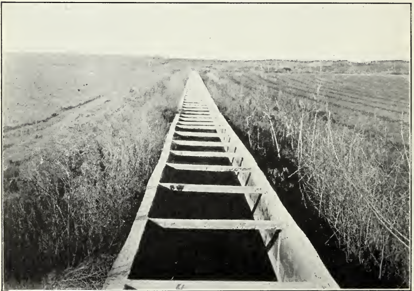
FIG. 2.—FLUME OR CHUTE CARRYING LONG POND WATER TO THE LARIMER AND WELD CANAL AND LINDENMEIER LAKE.
