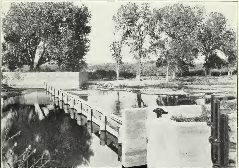
FIG. 2.—DIVERSION DAM OF THE B. H. EATON DITCH.
