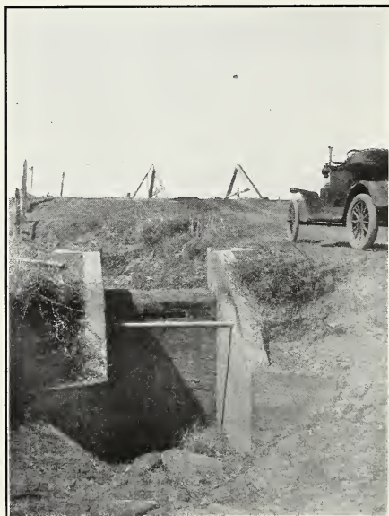
FIG. 2.—WEIR AND DROP AT THE HEAD OF THE CULVER-BARTELS LATERAL OF THE LARIMER COUNTY CANAL.
