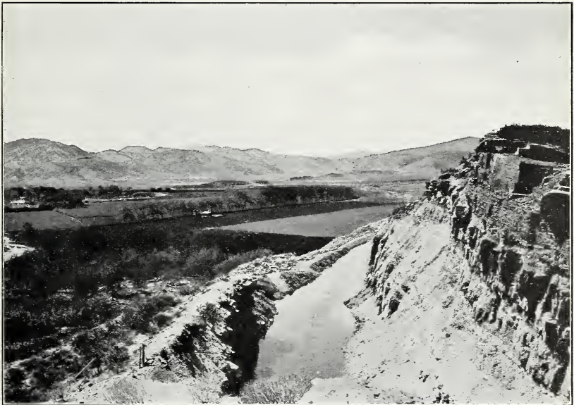
FIG. 2.—LINE OF THE POUDBRE VALLEY CANAL ROUNDING A ROCK BLUFF.
