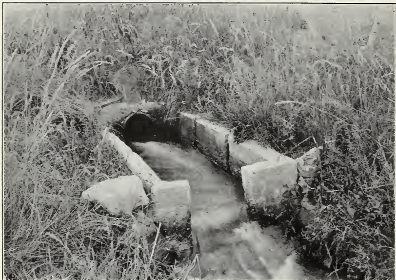
FIG. 1.—DEVICE FOR MEASURING WATER DELIVERED TO THE LATERALS OF THE PLEASANT VALLEY CANAL.
