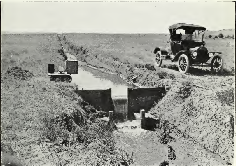
FIG. 2.—WEIR ON THE INLET OF THE DEALY RESERVOIR.
