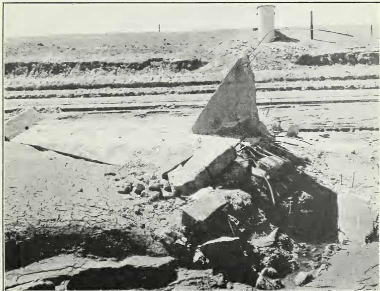
FIG. 2.—GATE TOWER BLASTED OUT AND REPLACED BY A WELL WITHIN THE DAM. NORTH POUDBRE RESERVOIR NO. 15.
