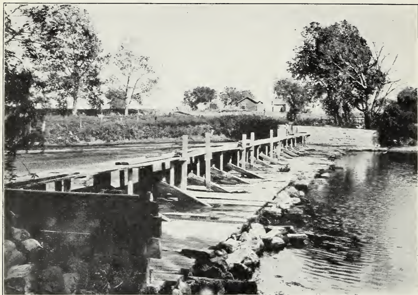
FIG. 1.—DIVERSION DAM OF THE GREELEY CANAL NO. 2.
