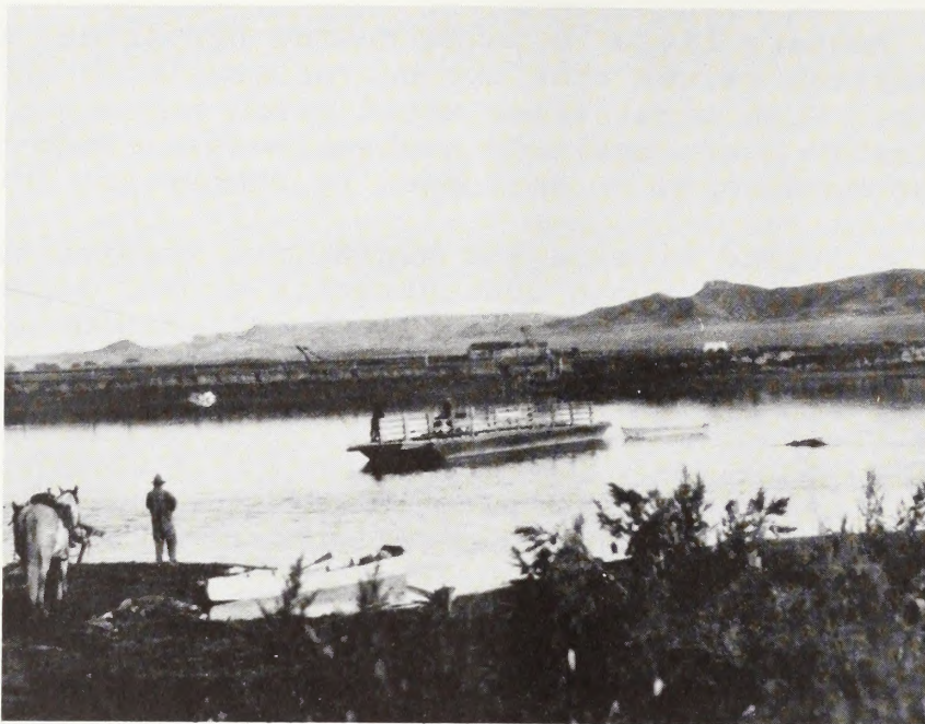
THE JUDITH FERRY ON THE MISSOURI RIVER HAS HISTORICALLY BEEN A MAJOR TRANSPORTATION LINK BETWEEN FERGUS AND CHOUTEAU COUNTIES. THE ORIGINAL FERRY APPEARS TO HAVE BEEN OPERATED BY USE OF A SWEEP AND THE RIVER'S CURRENT TO MOVE BETWEEN BANKS. (STANTON #940, n.d.)
