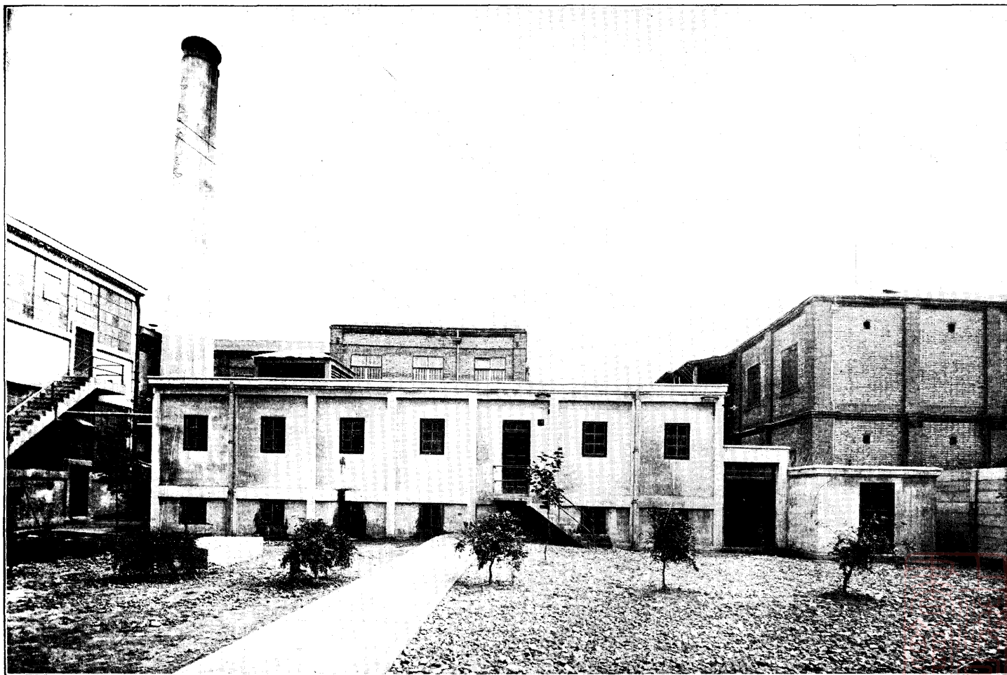
間子爐 BOILER HOUSE
