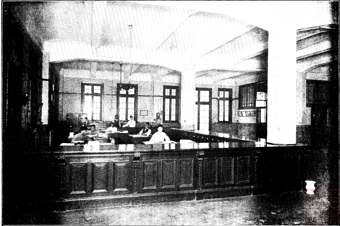
圖部內所務事 MAIN OFFICE
