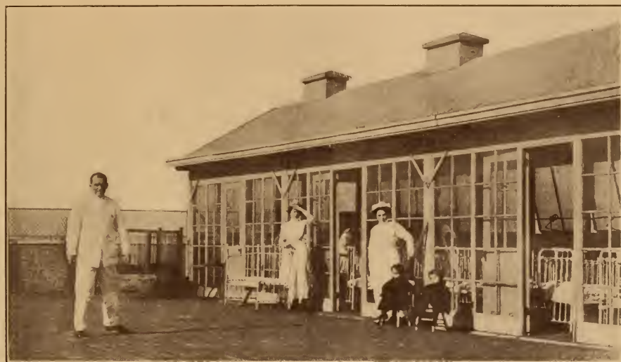
The New Roof Shelter.
