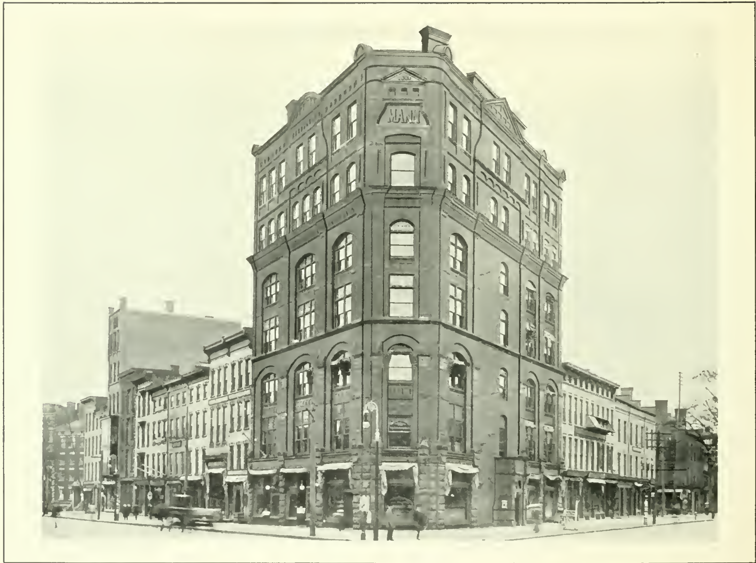
MANN BUILDING—GENESEE STREET, CORNER OF BROAD
