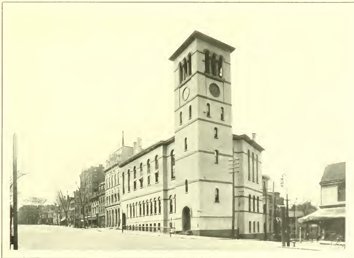
CITY HALL — GENESEE STREET, CORNER OF PEARL. Corner-stone laid in 1852
