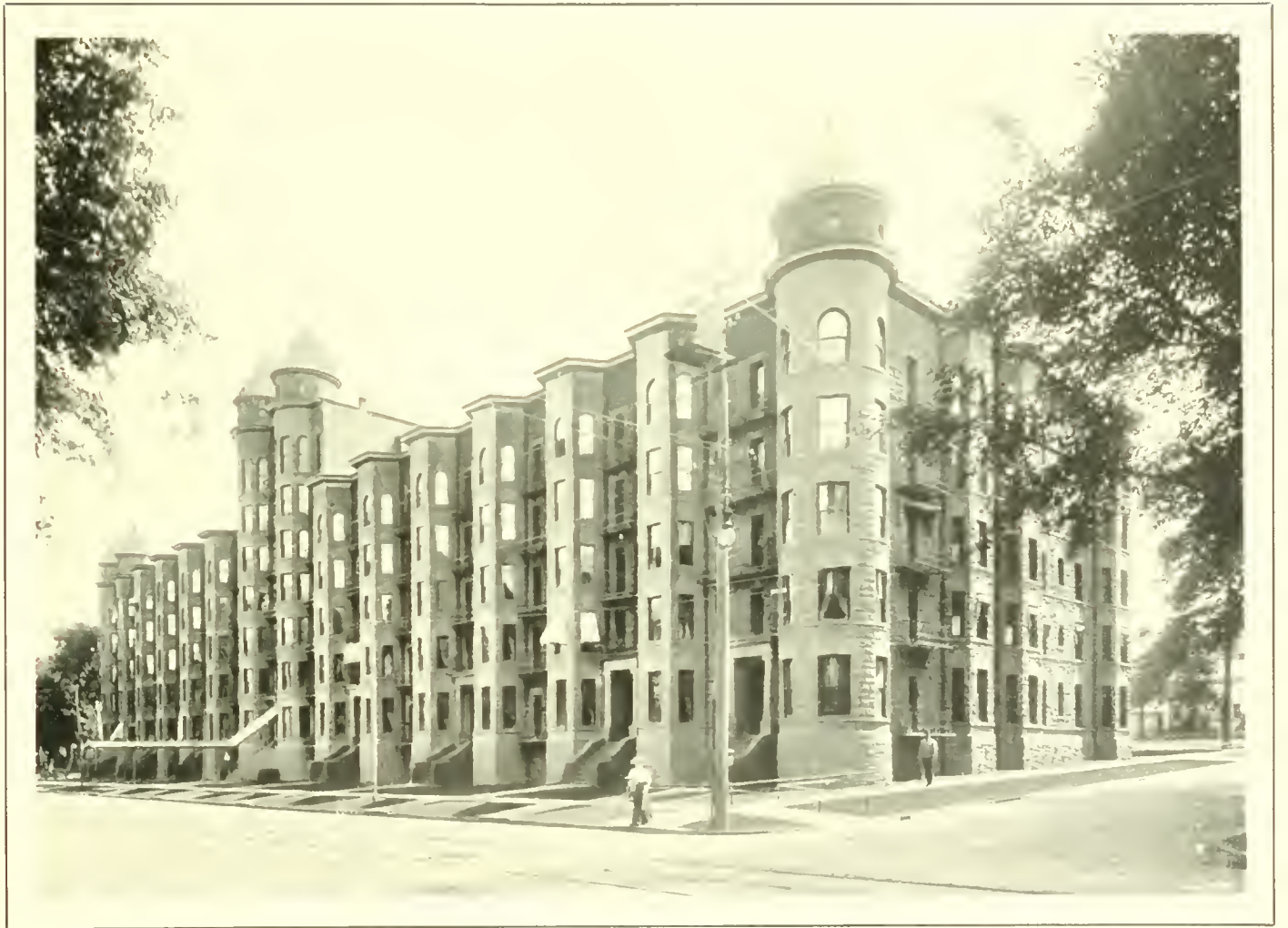
"THE OLBISTON" — GENESSEE STREET Containing 17 apartments
