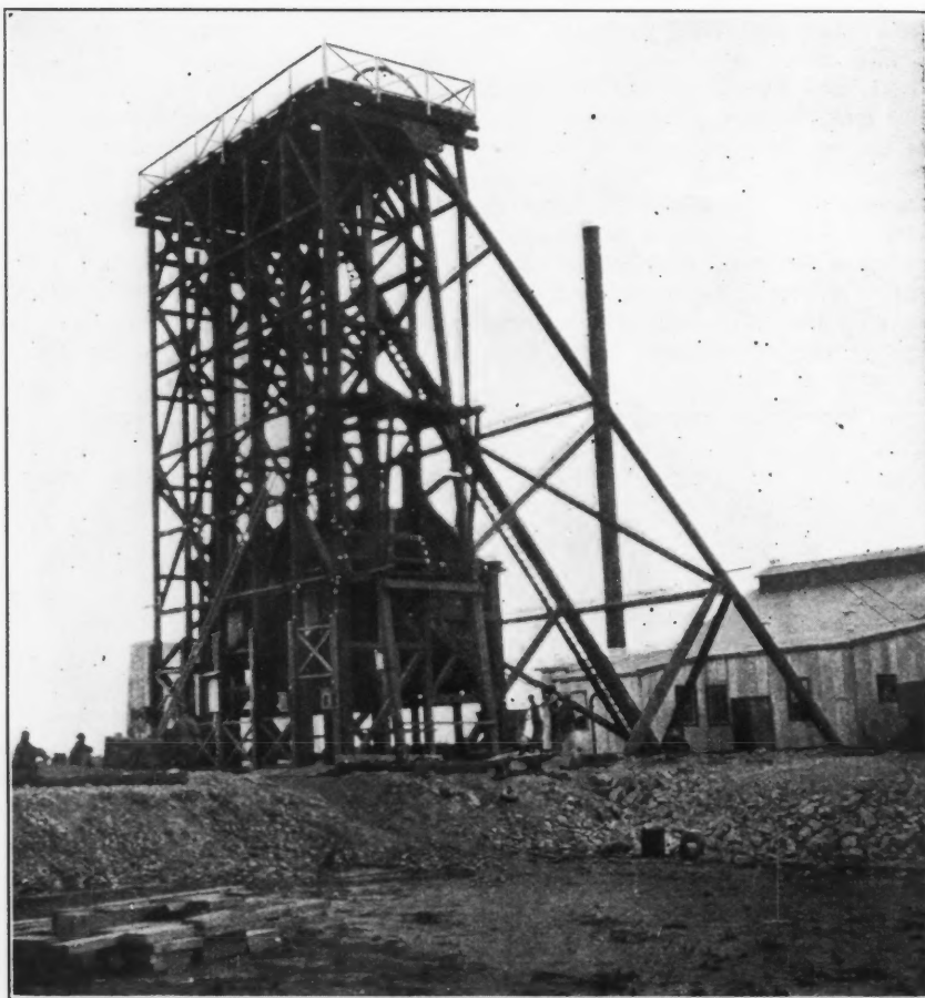
TEMPORARY, WOODEN HEADFRAME FOR SINKING SEVEN-COMPARTMENT SHAFT, APEX MINES, LTD.
