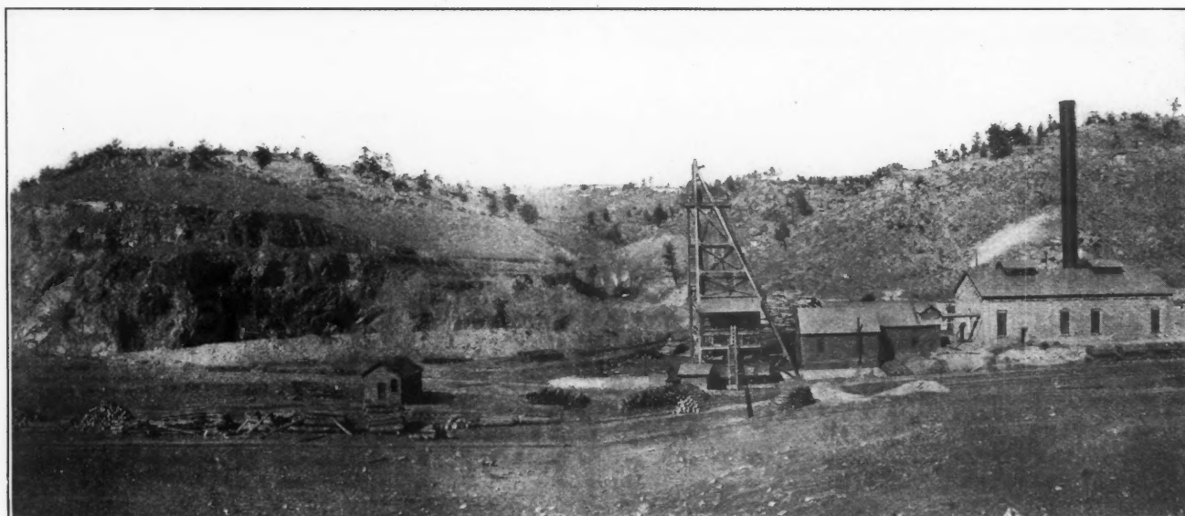
NORTH WALL OF PIT NO. 1, STEAM SHOVELS IN PIT NO. 2, AND STEEL HEAD FRAME AT MAIN SHAFT
