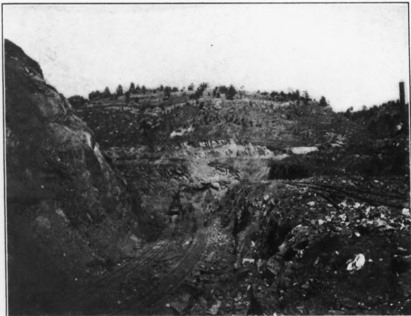
PIT NO. 1 UNDER STEAM SHOVEL OPERATION IN 1905
