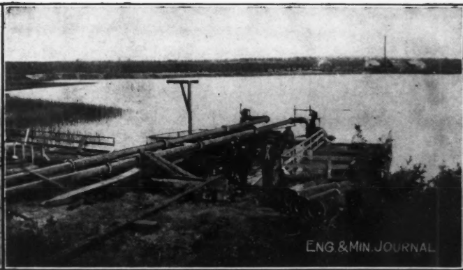
PUMPS, DISCHARGE AND RAFTS, CARSON LAKE
