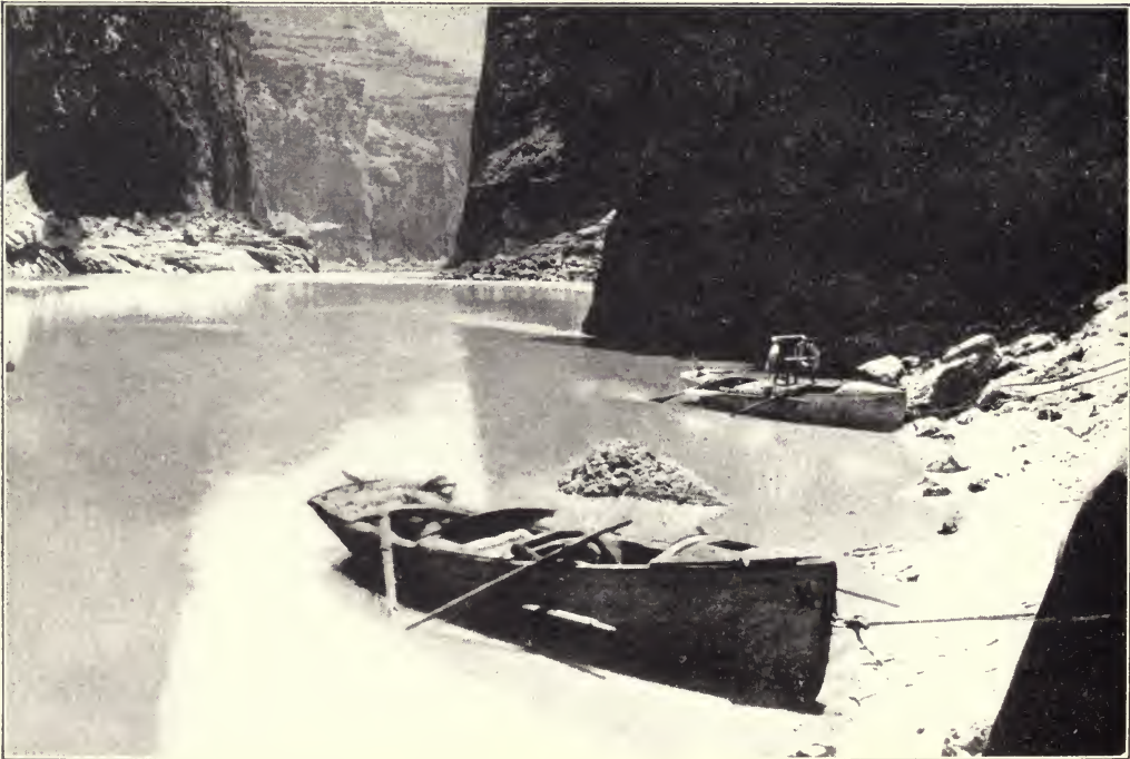
Photograph by U. S. Geological Survey
