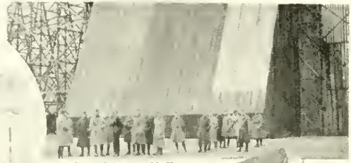
Door of the Dirigible Hangar Near Camp
