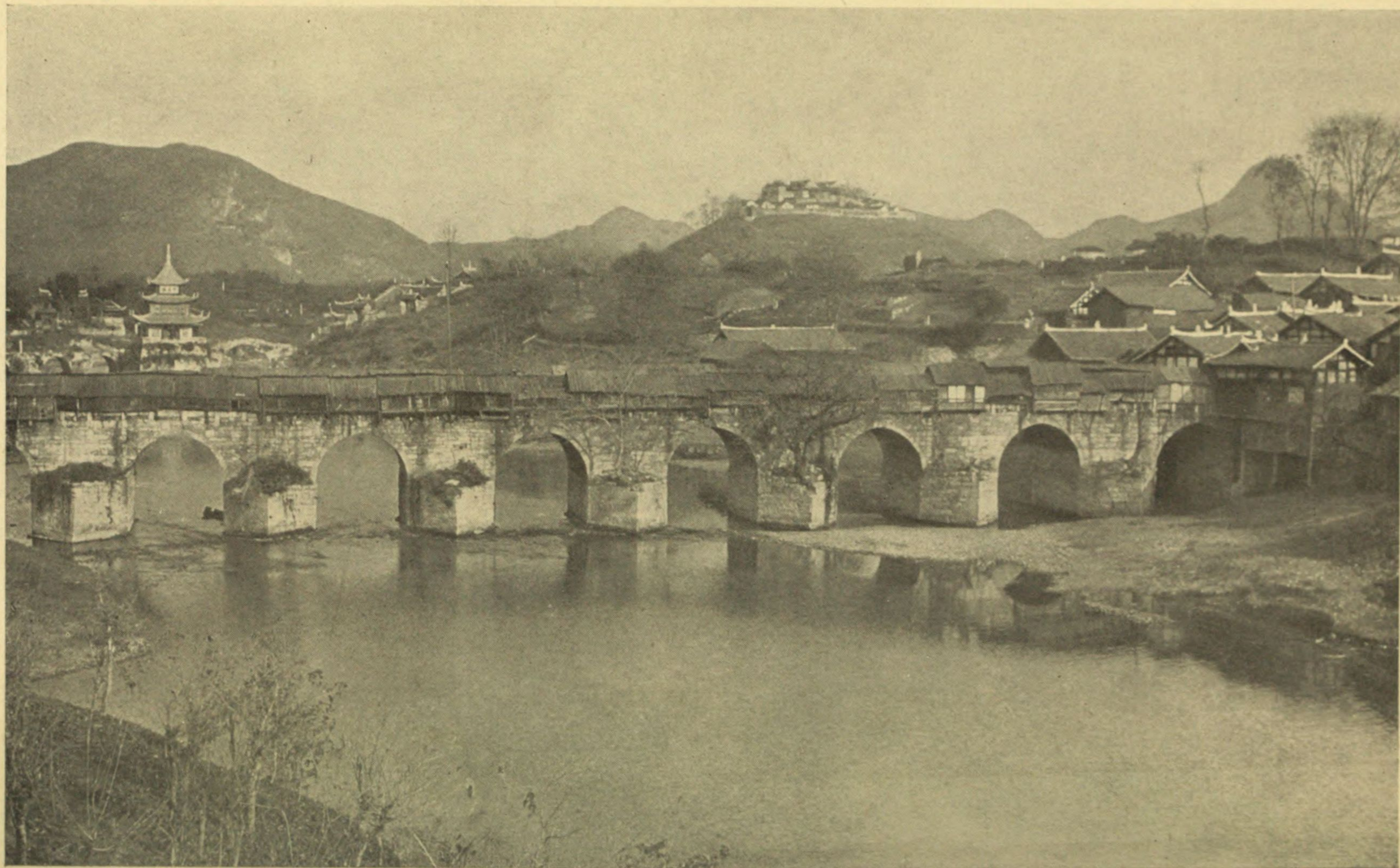
THE BEAUTIFUL BIG SOUTH BRIDGE, REMOTE KWEIYANG.
