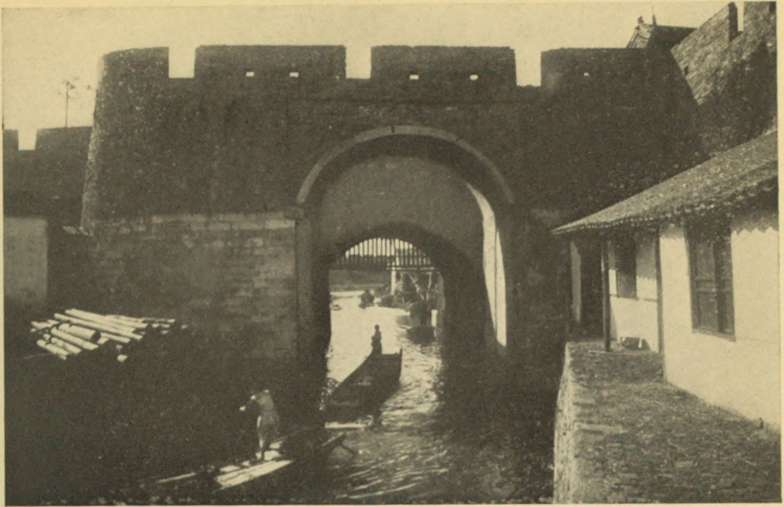
SOO'S SOUTH (WATER) GATE. The City has five such gates, beautiful and interesting.
