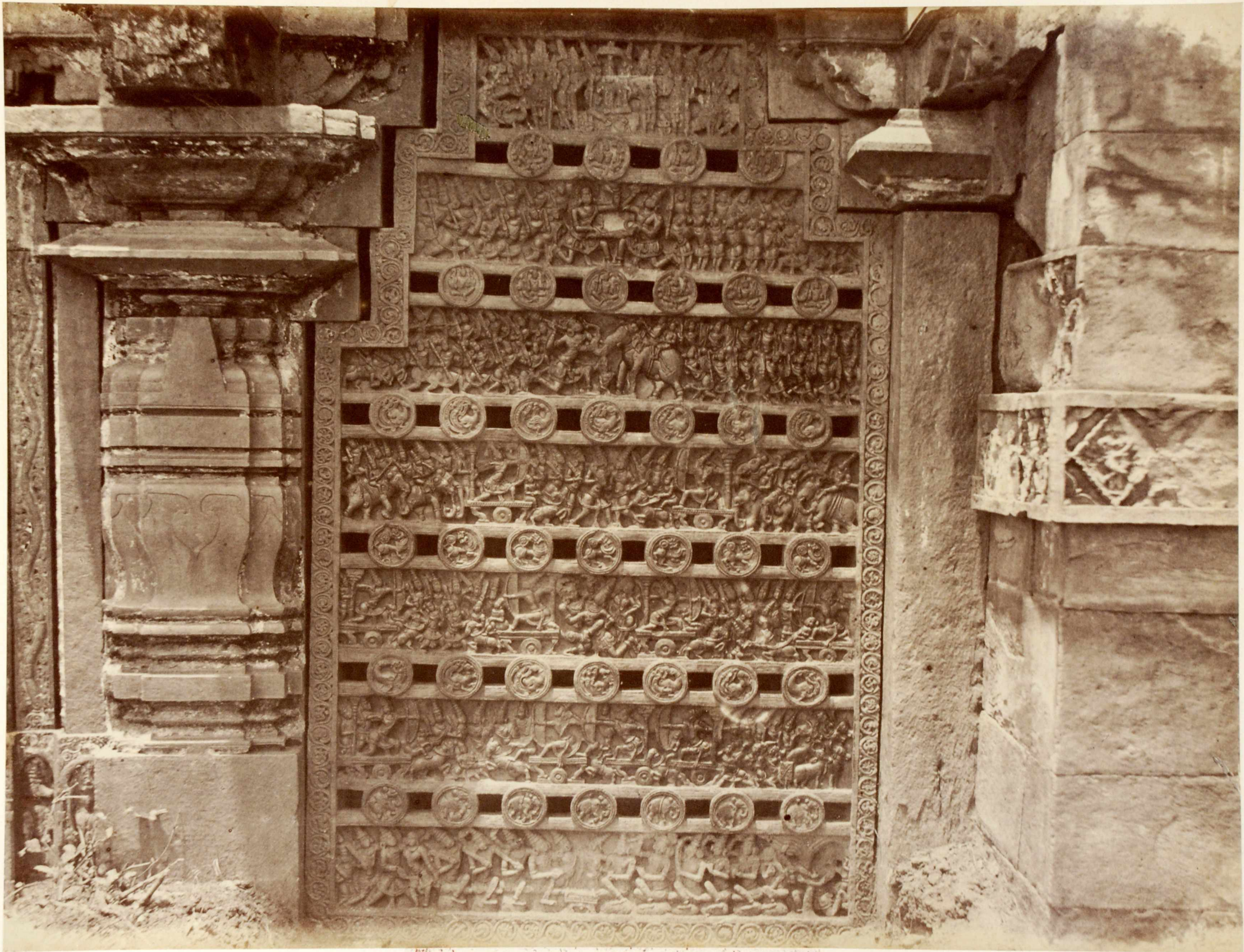
PLATE LI. NURSAPOOR. Window of perforated Stone.
