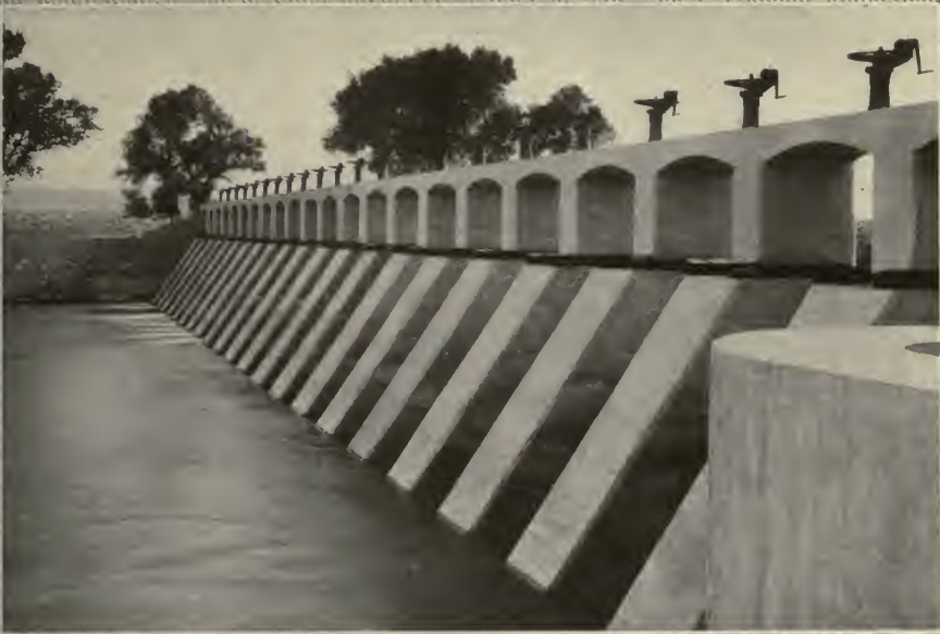
MAIN DAM ON THE TRUCKEE IRRIGATION DITCH
