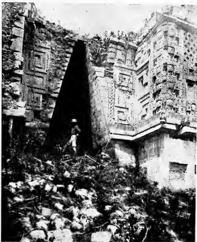
Plate XV. A Sealed Portal Vault in the House of the Governor at Uxmal. The veneer character of the cut stone comes out clearly. Peabody Museum photograph.
