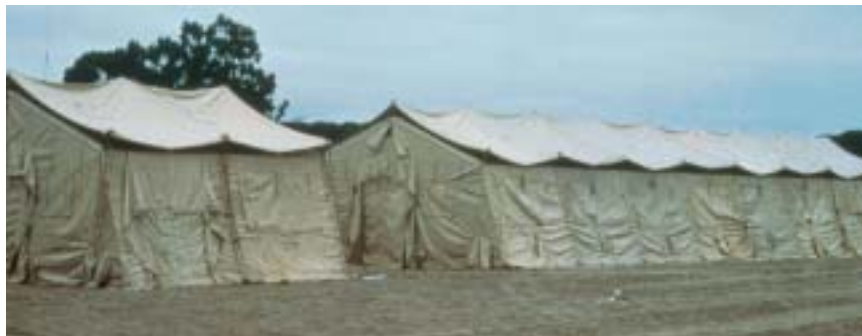
Fig. 6-7. Two TEMPER tent modules have been combined to form the tent on the left, while eight modules have been combined to form the tent shown in the rear. TEMPER: tents, extendable, modular, personnel.
