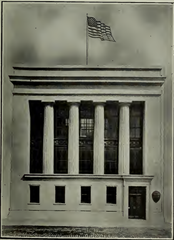
BALFOUR-GUTHRIE BUILDING L. B. Dutton, Architect.
