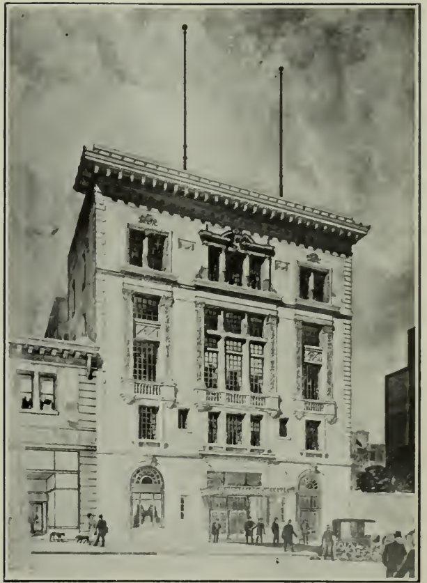
KNIGHTS OF COLUMBUS BUILDING Smith O'Brien, Architect.
