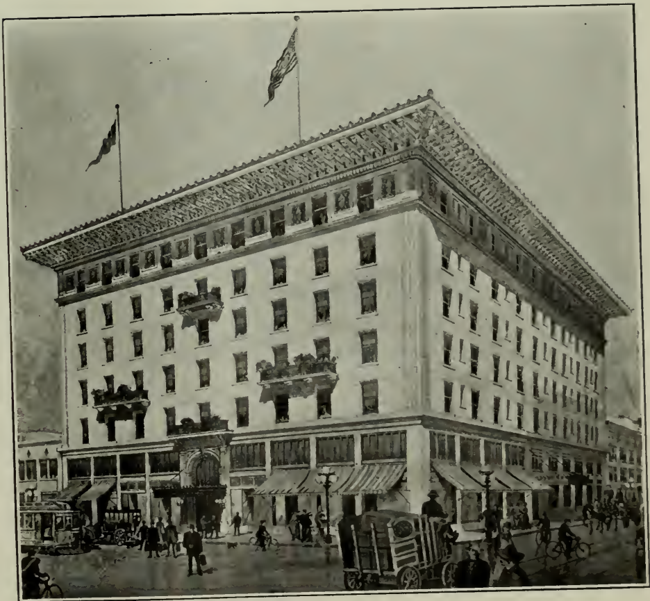
NEW COMMERCIAL HOTEL BUILDING Fresno, Calif.
