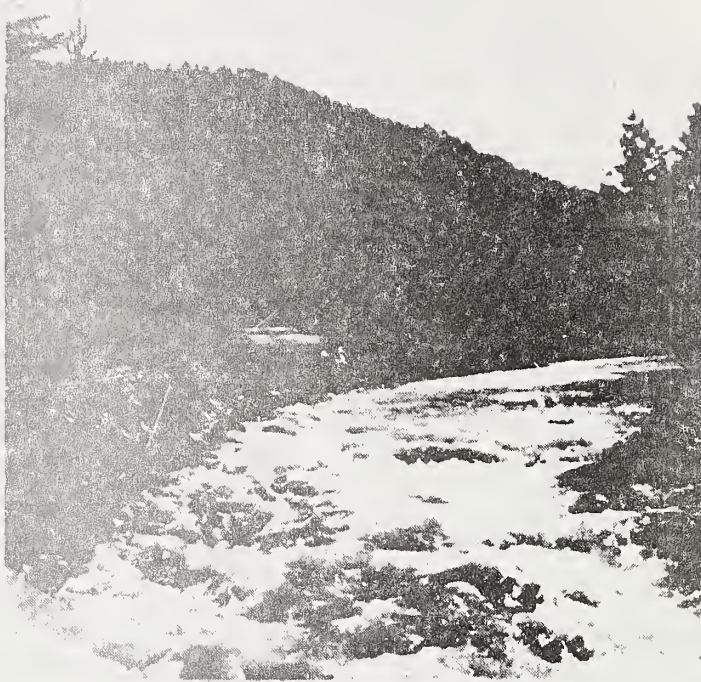
END OF THE ROAD AFTER THE 1973 FLOOD
