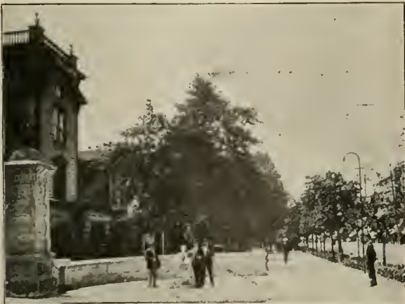
HOT WATER FOUNTAIN ON BATHHOUSE ROW.
