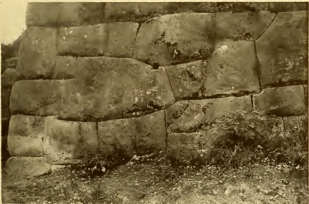
FIG. 72.—A portion of a wall in the great Inca fortress near Cuzco. The stones are fitted with great exactness, but without mortar. A drainage opening is shown in center. The corner stones are rounded and the wall slopes a little. The Incas had no beasts of burden (the llama will carry 75 pounds, but will not pull in harness) and no metal tools. Some of the large stones weigh many tons.
