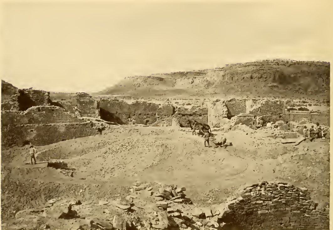
FIG. 88.—In excavating the central portion of Pueblo del Arroyo, debris from the individual rooms was wheeled in barrows to accessible points and dragged thence to an elevated trap through which it was poured into steel tram cars. (Photograph by O. C. Havens. Courtesy of the National Geographic Society.)
