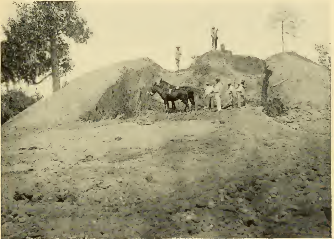
FIG. 243.—Marksville. Trench partly excavated, Mound 4.
