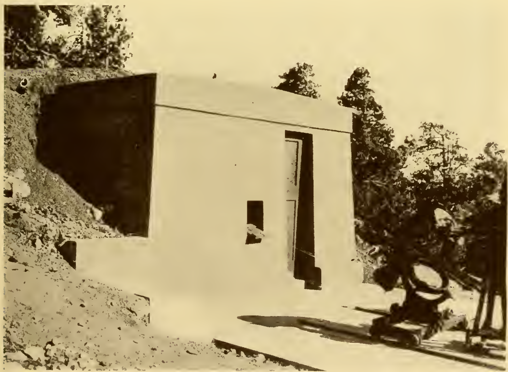
FIG. 32.—Concrete observing tunnel at Table Mountain, California.
