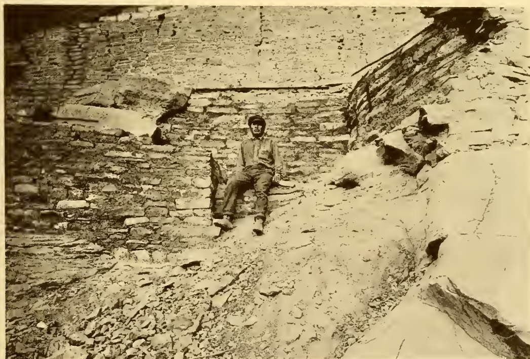
FIG. 121.—New foundation of Tower from in front. All masonry below dark lines is portion of repair work.
