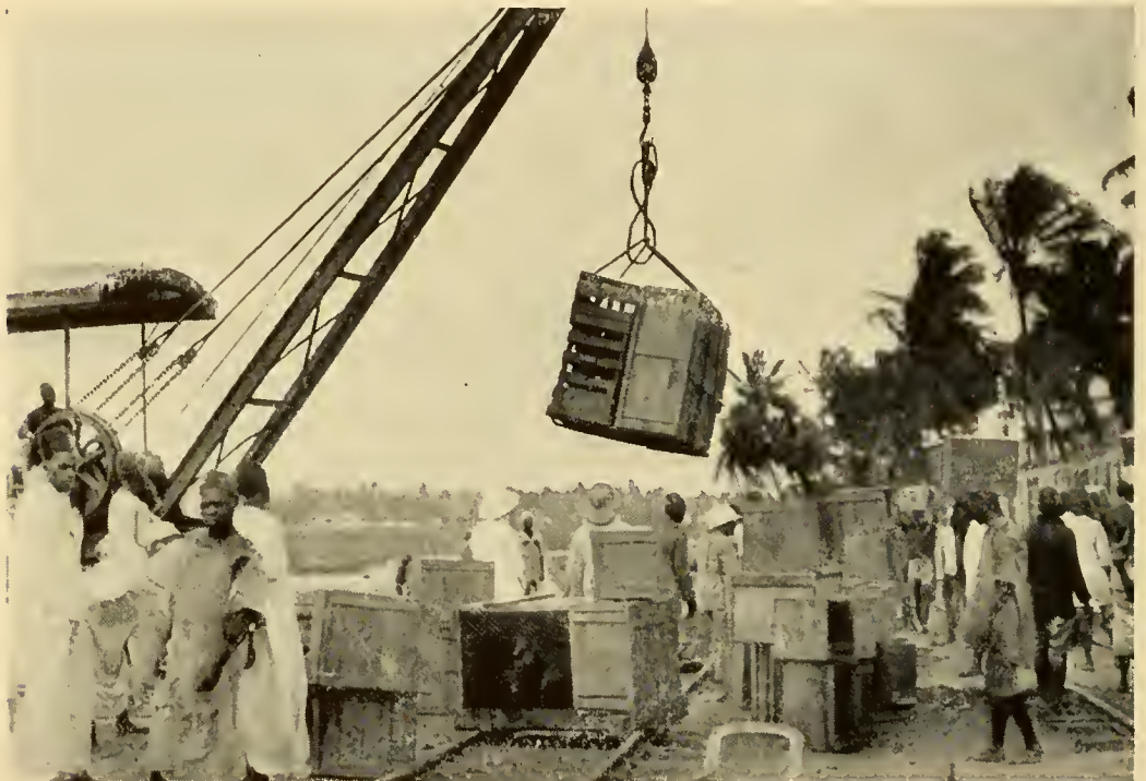
FIG. 25.—Handling stock at Dar-es-Salaam.
