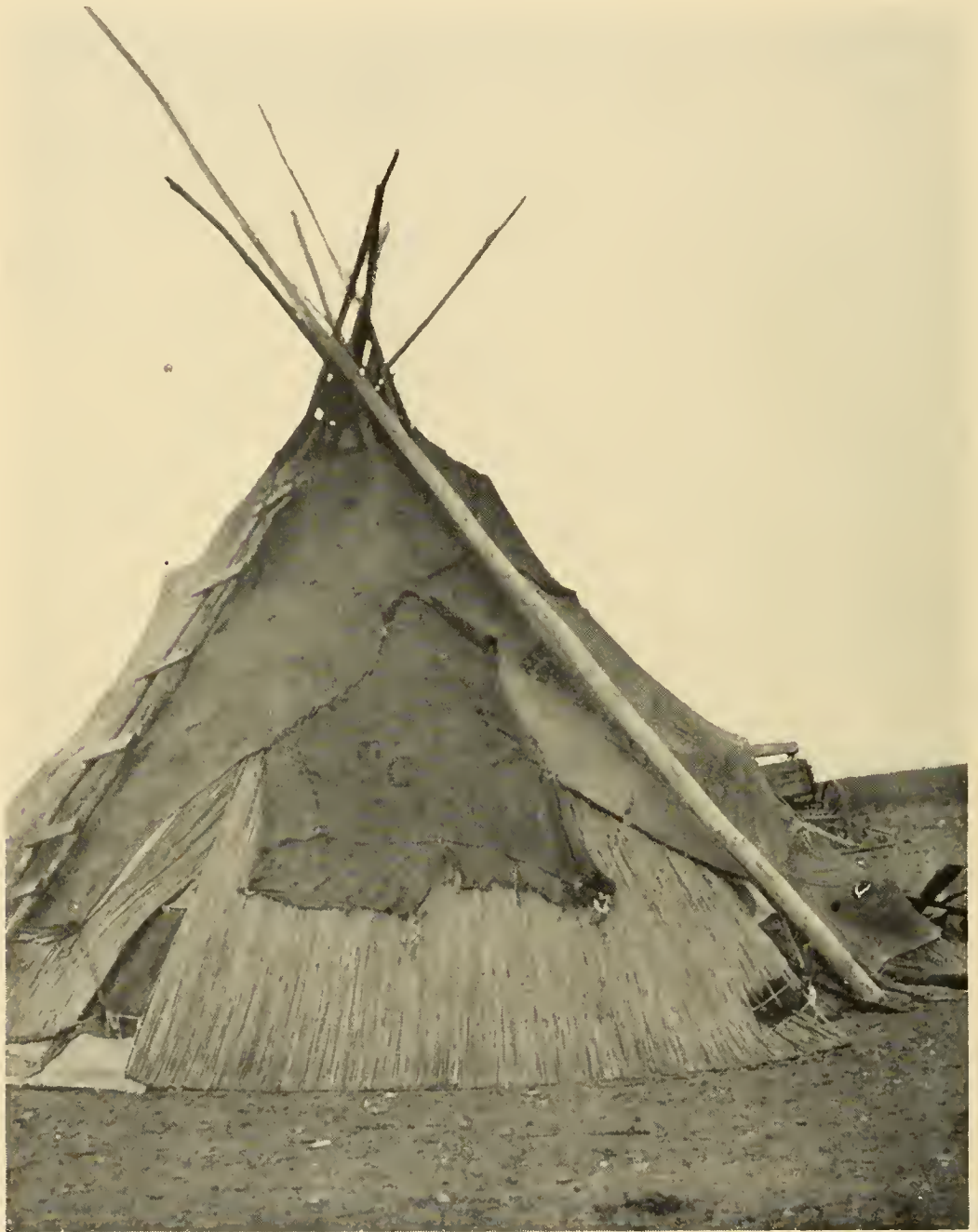
FIG. 193.—Tipi used by the Wanapum or Columbia River Indians at the Lower Falls of the Yakima River, Benton County, Washington. The habitation is a temporary one and is constructed of tule reeds covered with skins and burlap. The old type of semisubterranean pit house was abandoned before the time of the Lewis and Clark expedition.
