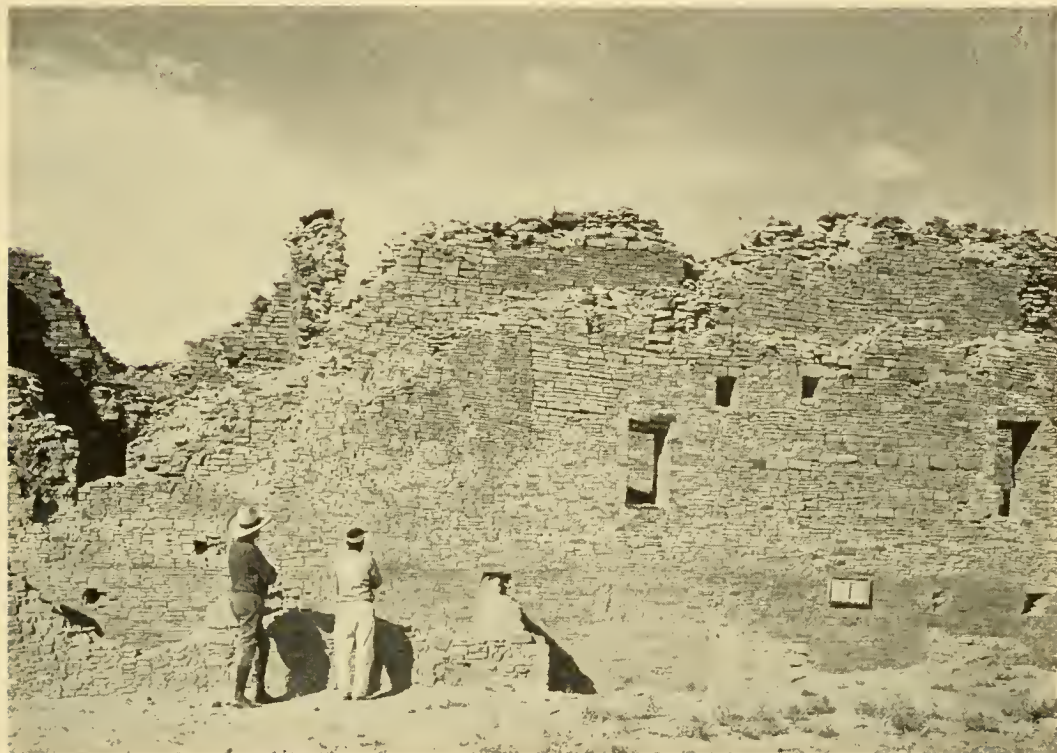
FIG. 166.—Outer south wall of Pueblo del Arroyo, showing varied stonework and later, abutting rooms. (Photograph by Neil M. Judd. Courtesy of the National Geographic Society.)
