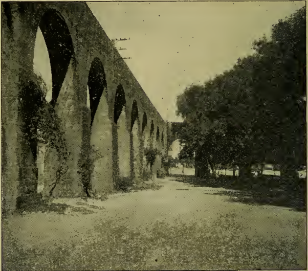
THE AQUEDUCT, MORELIA.
