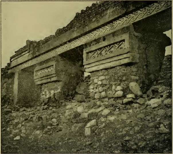
A CRUMBLING WALL.
