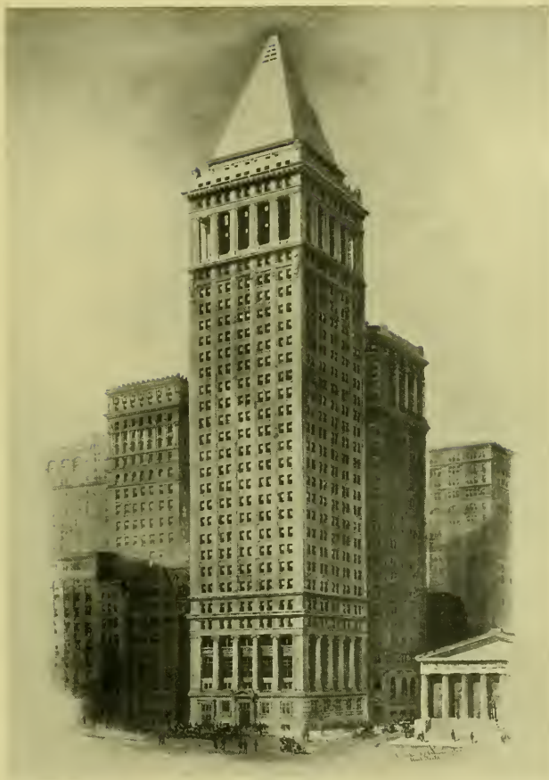
The Bankers Trust Building, Wall and Nassau Streets
