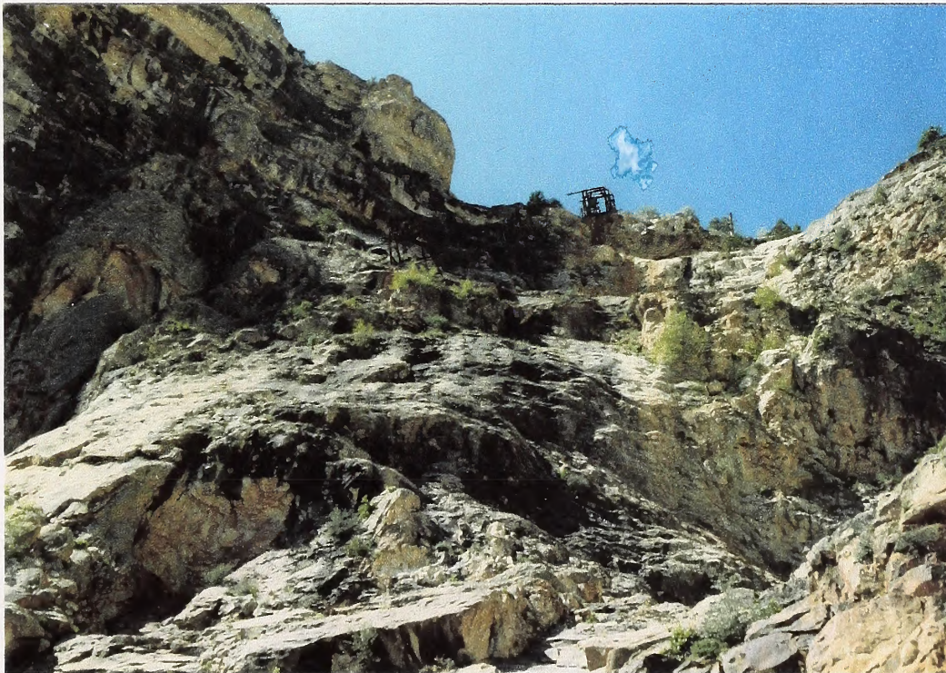
PHOTO #9: A view of the two intermediate aerial tramway towers from the lower adit area.
