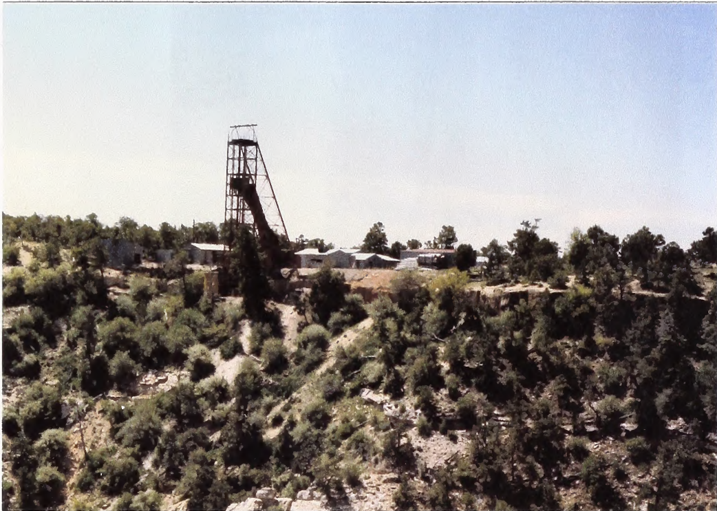
PHOTO #1: The view of the Orphan Mine facilities located on the South Rim of the Grand Canyon. The photo is taken from the Powell Memorial.
