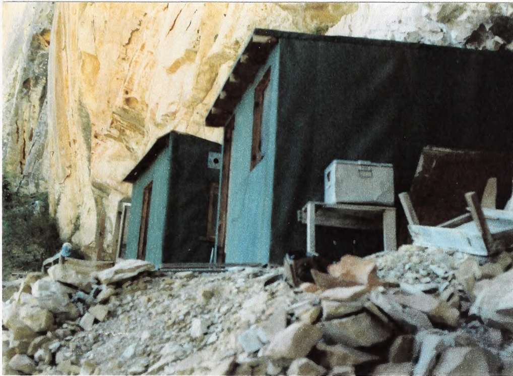
PHOTO #6: A view of the bunkhouses located at the lower adit area of the Orphan Mine. The ledge that these structures sit on is located at the left of top center of Photo #4.
