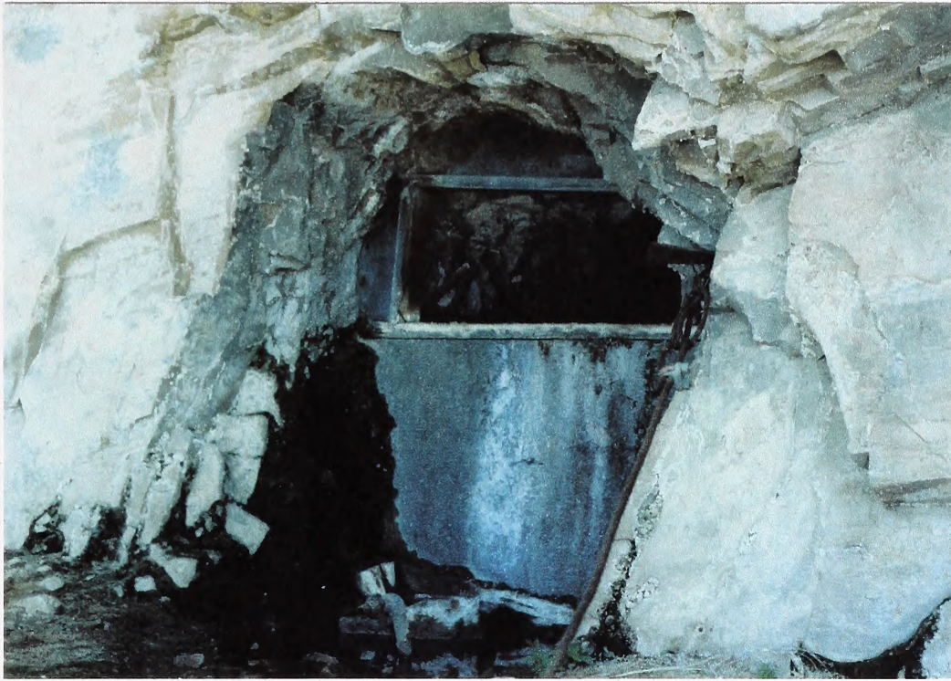
PHOTO #8: A closer view of the partially bulkheaded adit seen in Photo #7.
