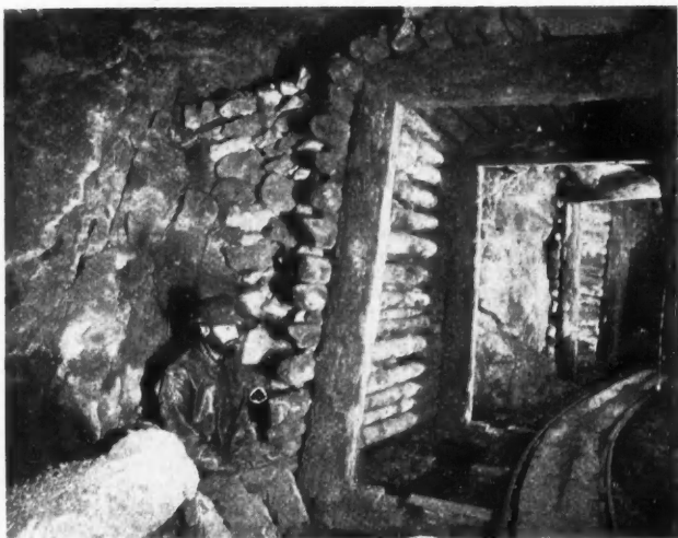
TIMBERING AT CURVE.
