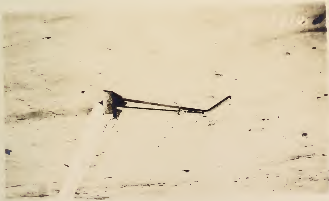
FIG. 2A - CENTER-LINE GROOVE TAMPER MOUNTED ON A 2 INCH X 6 INCH X 12 FOOT PLANK. BOTH ENDS OF THE TOOL ARE CONSTRUCTED IDENTICALLY THE SAME.
