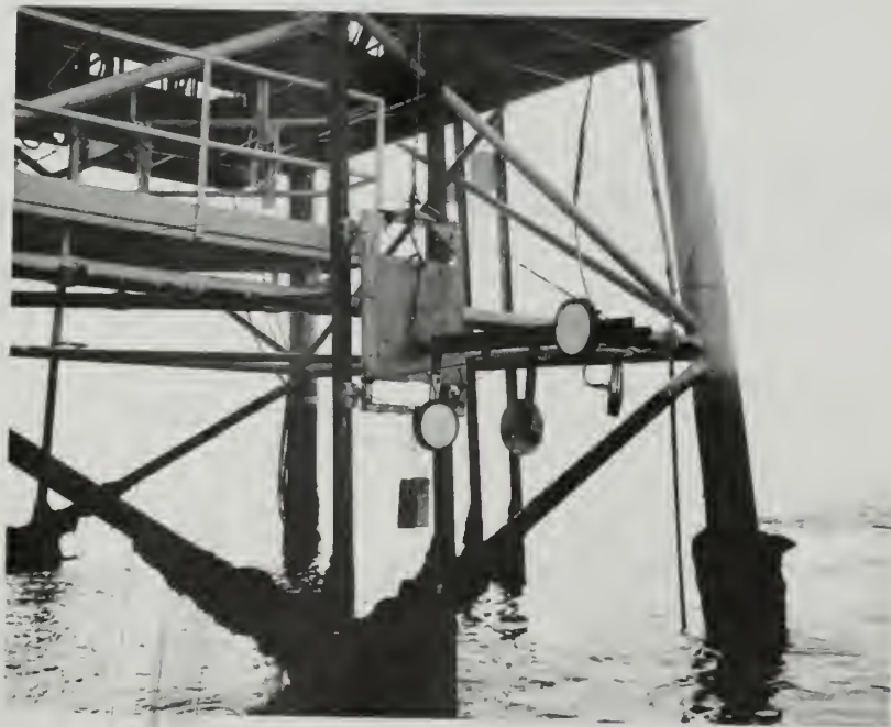
TRANSDUCER ASSEMBLY INSTALLED, N.E.L. TOWER
