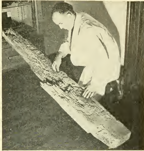
FIG. 67 A beam of wood almost completely destroyed by termites. What can be done to prevent damage to wood by termites? (SCIENCE SERVICE)
