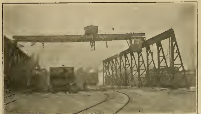
FIG. 6—ASH PITS AND TRAVELLING CRANE.
