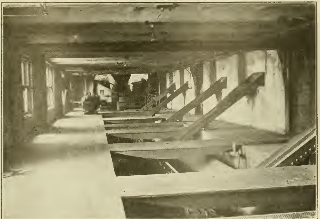
BASEMENT OF BOILER ROOM SHOWING COAL AND ASH CONVEYER.
