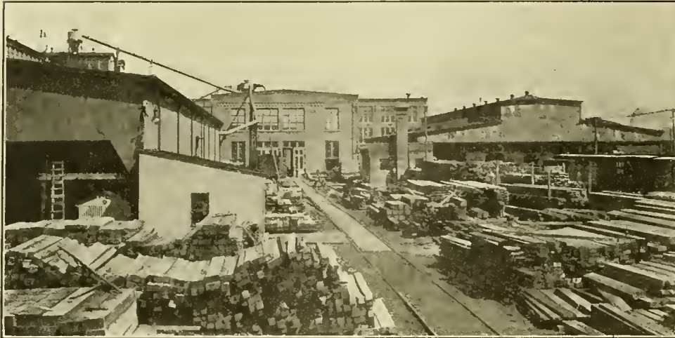
LOOKING NORTH FROM SILL YARD—LUMBER SHED TO THE LEFT, PLANING MILL IN CENTER, FREIGHT CAR SHOP TO THE RIGHT.
