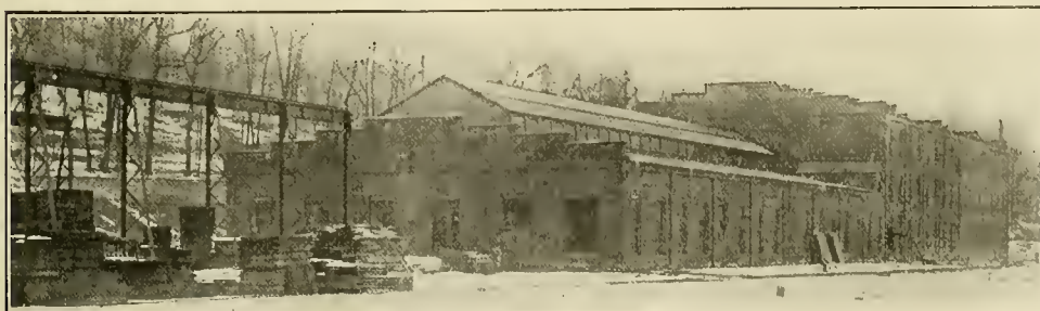
PATTERN SHOP AND PATTERN STORAGE BUILDING.
