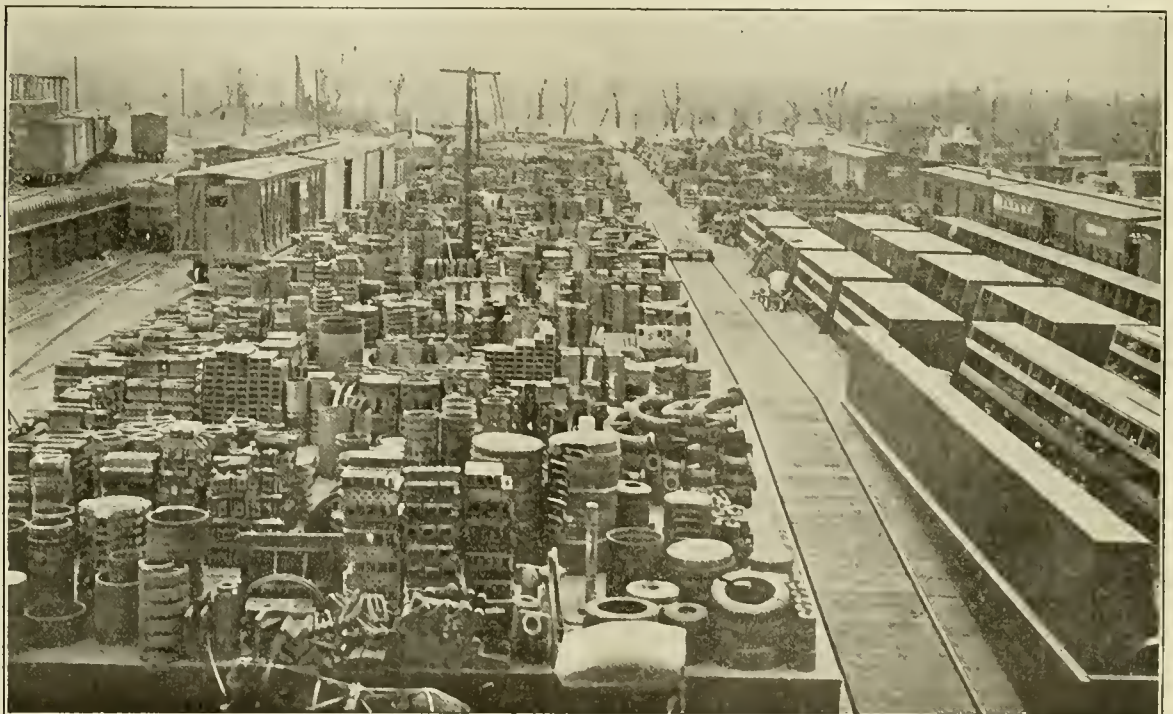
FIG. 28.—FINISHED MATERIAL PLATFORM, TOPEKA STOREHOUSE.
