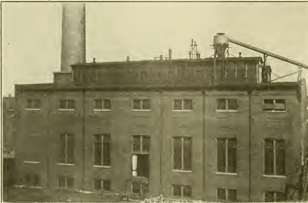
POWER HOUSE—VIEW FROM TOP OF LUMBER SHED.
