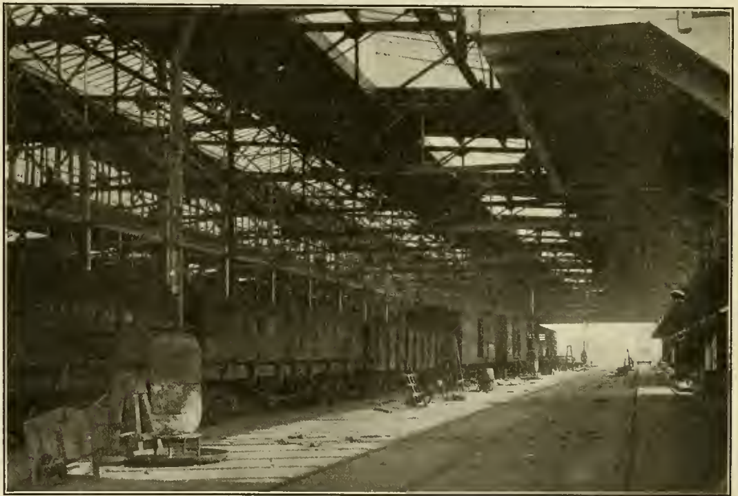
INTERIOR OF NEW FREIGHT CAR SHOP.
