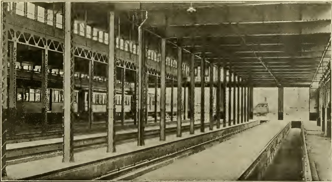
INTERIOR OF INSPECTION SHED AT DUNTON—LONG ISLAND RAILROAD.
