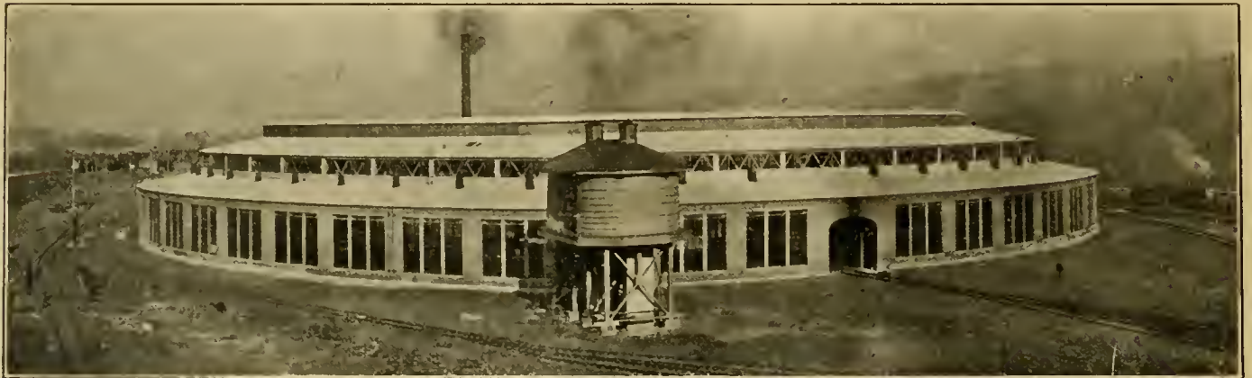
FIG. 2—ROUNDHOUSE, SHOWING TWO OF THE STORAGE TRACKS AT THE LEFT.
