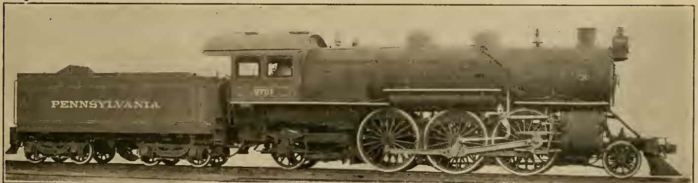
PRAIRIE (2-6-2) TYPE PASSENGER LOCOMOTIVE, WITH WALSCHAERT VALVE GEAR—PENNSYLVANIA RAILROAD.
