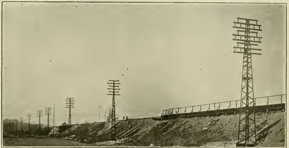
STEEL POLES AND TRANSMISSION LINES—LONG ISLAND R. R.
