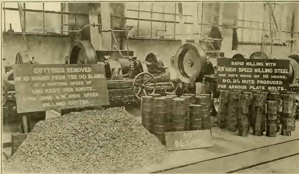
MAKING HEXAGON NUTS FROM ROLLED BARS.
