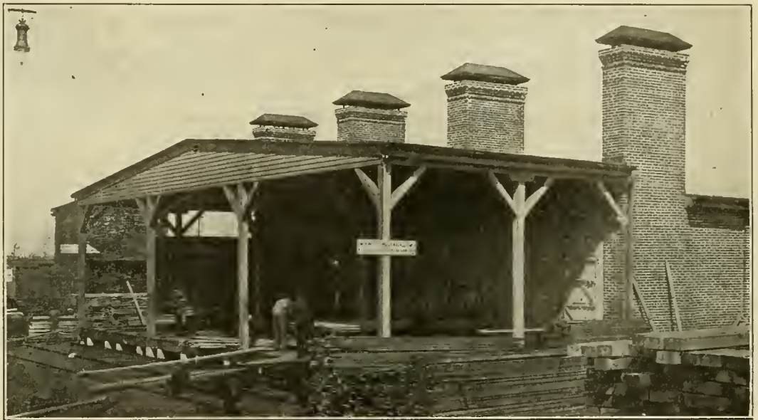
RECEIVING PLATFORM OF DRY KILN.
