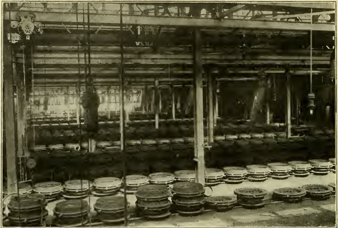
MOULDING FLOOR, SOUTH ALTOONA WHEEL FOUNDRY.
