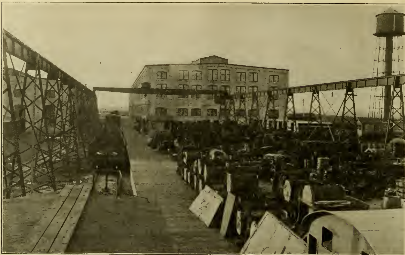
STOREHOUSE, STORAGE PLATFORM AND TRAVLING CRANE.
