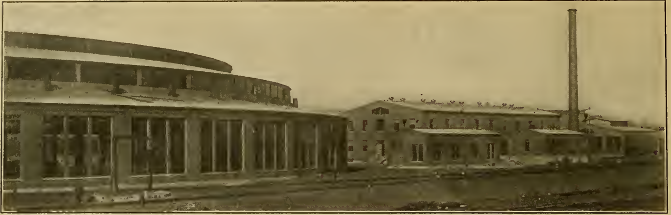
FIG. 17.—PART OF THE ROUNDHOUSE WITH THE OFFICE BUILDING, POWER PLANT, FAN HOUSE AND OIL HOUSE TO THE RIGHT (FAN HOUSE HAS SINCE BEEN CONNECTED TO THE ROUNDHOUSE.)
