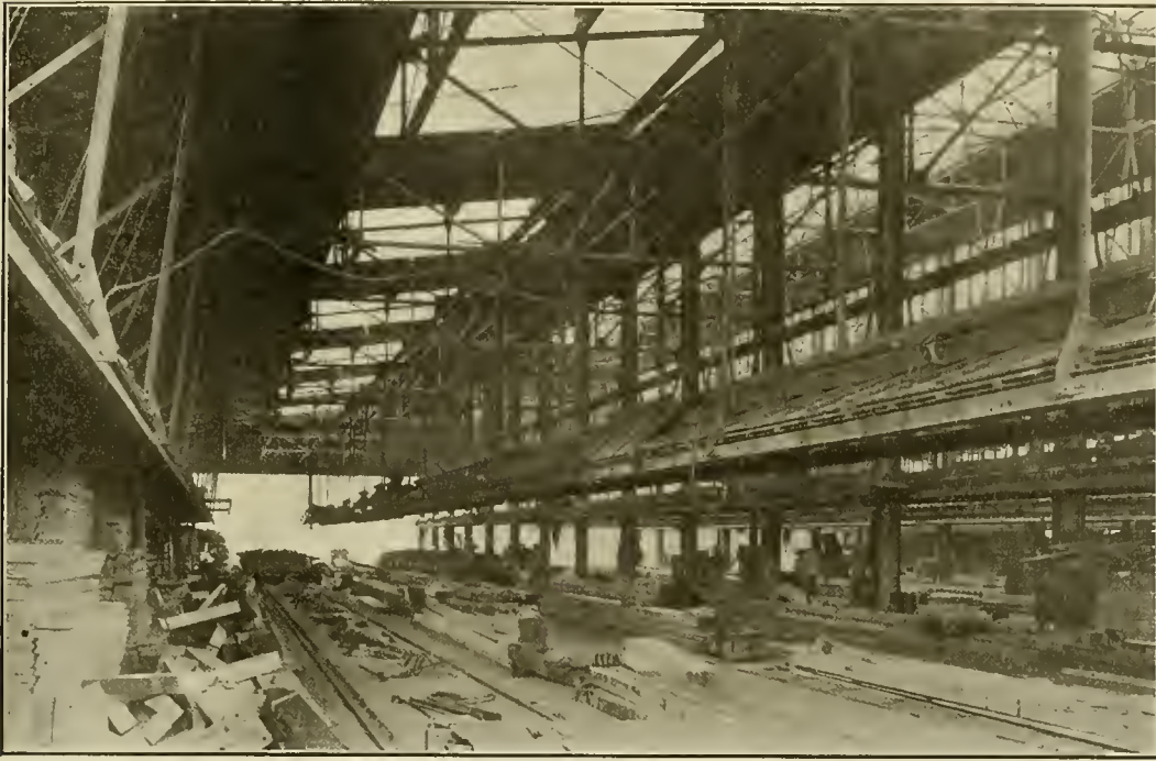
INTERIOR OF FREIGHT CAR REPAIR SHOP.
