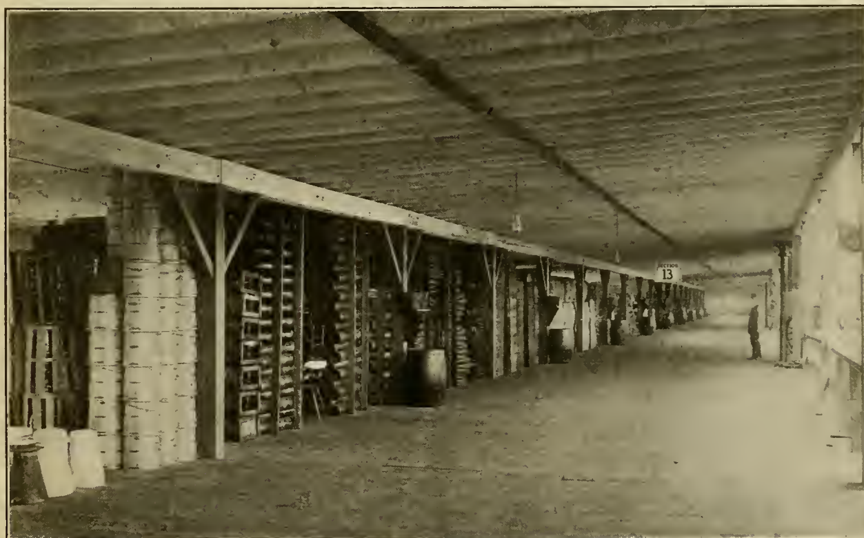
SECTION 13, SECOND FLOOR—EAST MOLINE STOREHOUSE.
