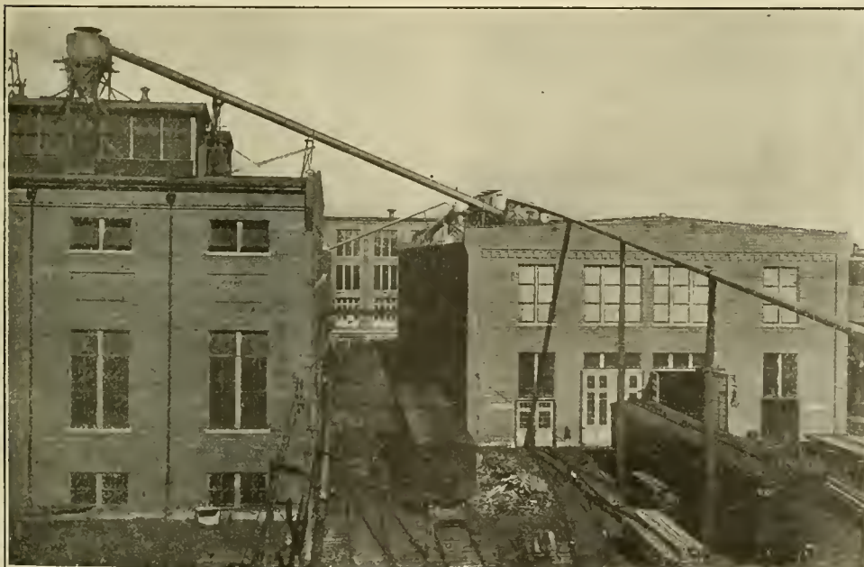
PLANING MILL, SHOWING SHAVING EXHAUST PIPE EXTENDING TO THE ROOF OF THE POWER HOUSE.
