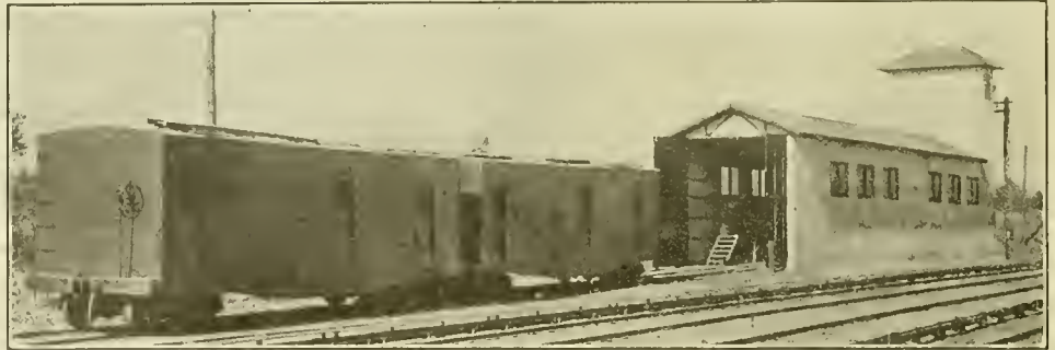
PORTABLE SUB-STATION AND HOUSE—J. I. R. R.
