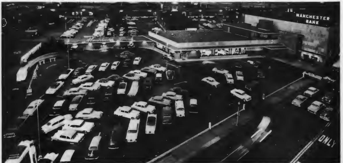
Drive-up and parking facilities, Manchester Bank, St. Louis, where some 3,000 transactions per day are handled
